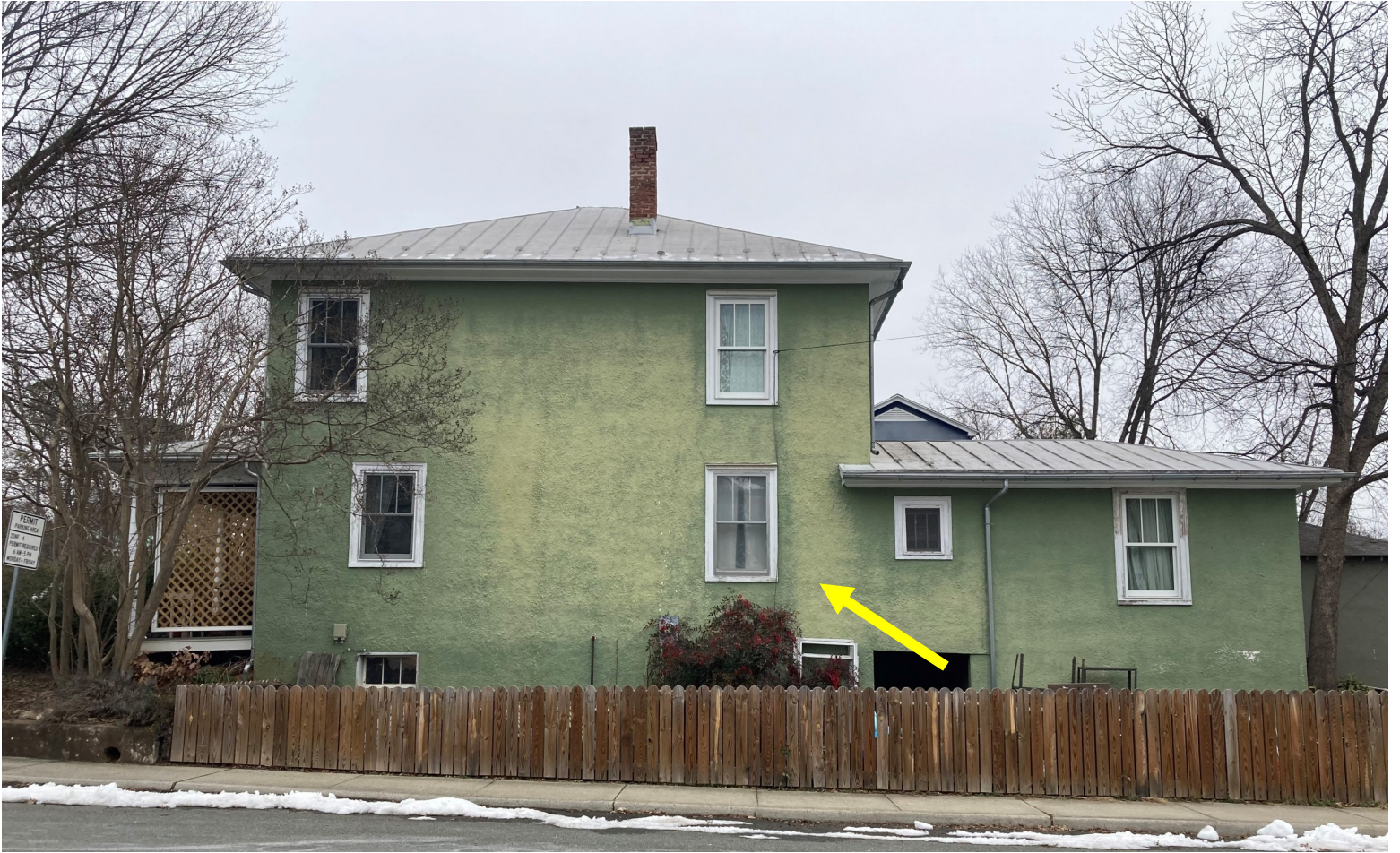
600 Lexington Avenue — Window replacement, south elevation — BAR review Feb 22, 2023
