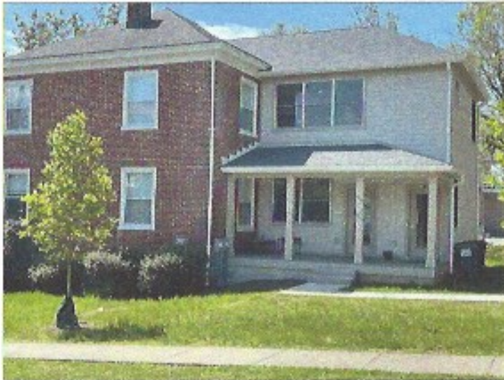
SIDE OF RESIDENCE FROM GRODON AVENUE
