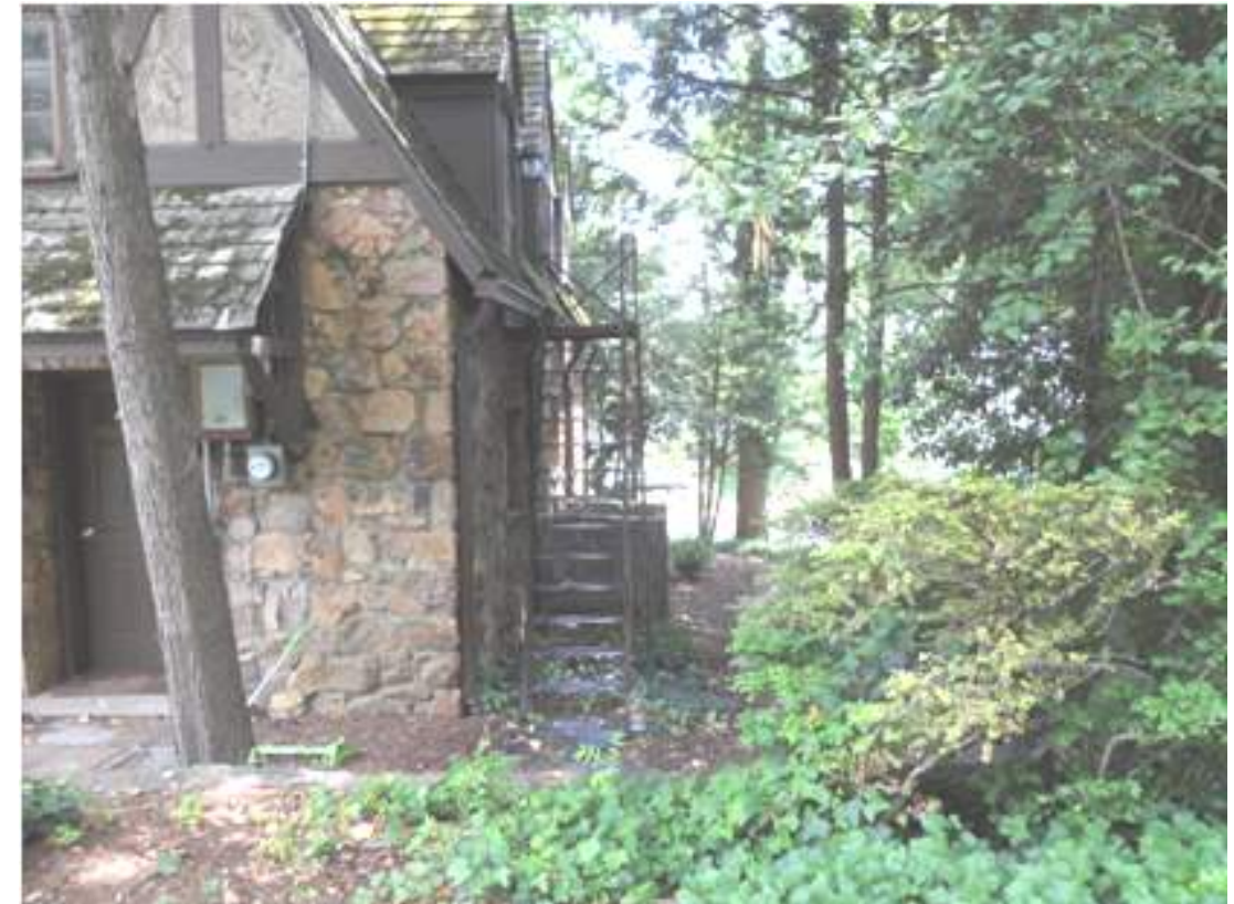
METAL FIRE ESCAPE
