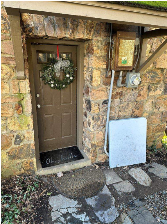
New front door w/ bracketed roof
