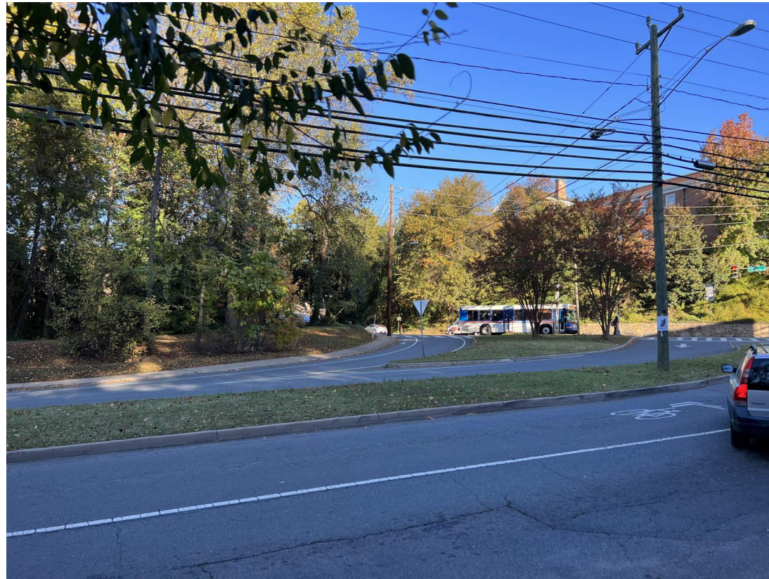
JEFFERSON PARK AVENUE - LOOKING NORTH
