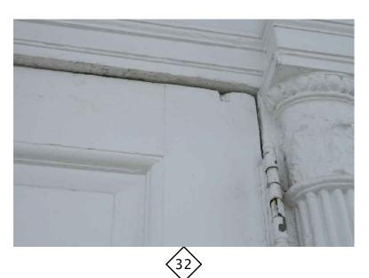
WATER CONTROL: CONFIRM WATER-TIGHT JOINTS UNDER PILASTER AND WALL AND INSTALL MORTAR DAM AT LEFT TO DIVERT WATER AWAY FROM FACE OF BRICK WALL. SEAL ALL WALL PENETRATIONS WITH EXPANDABLE FOAM, FLEXIBLE GASKETS OR MORTAR AS NECESSARY TO CLOSE UP GAPS AROUND PIPES, WIRES, ETC.
