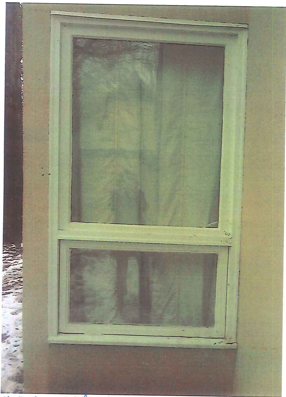
North-facing window to be replaced
