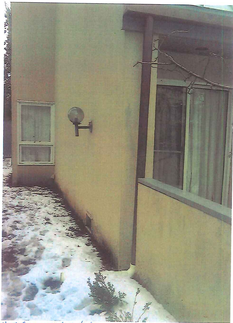
North-facing window to be replaced
