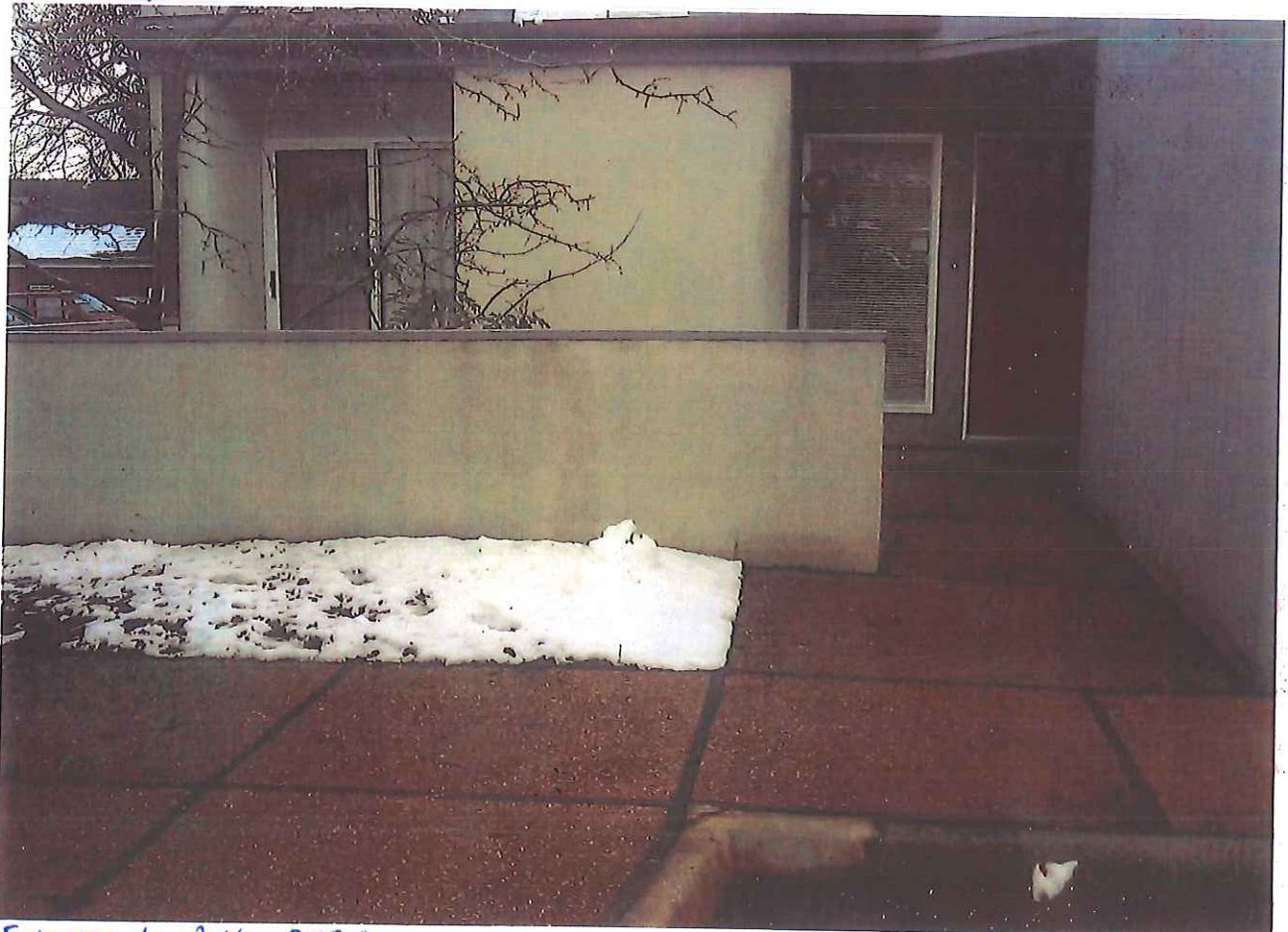
Entrance to Unit 203A
