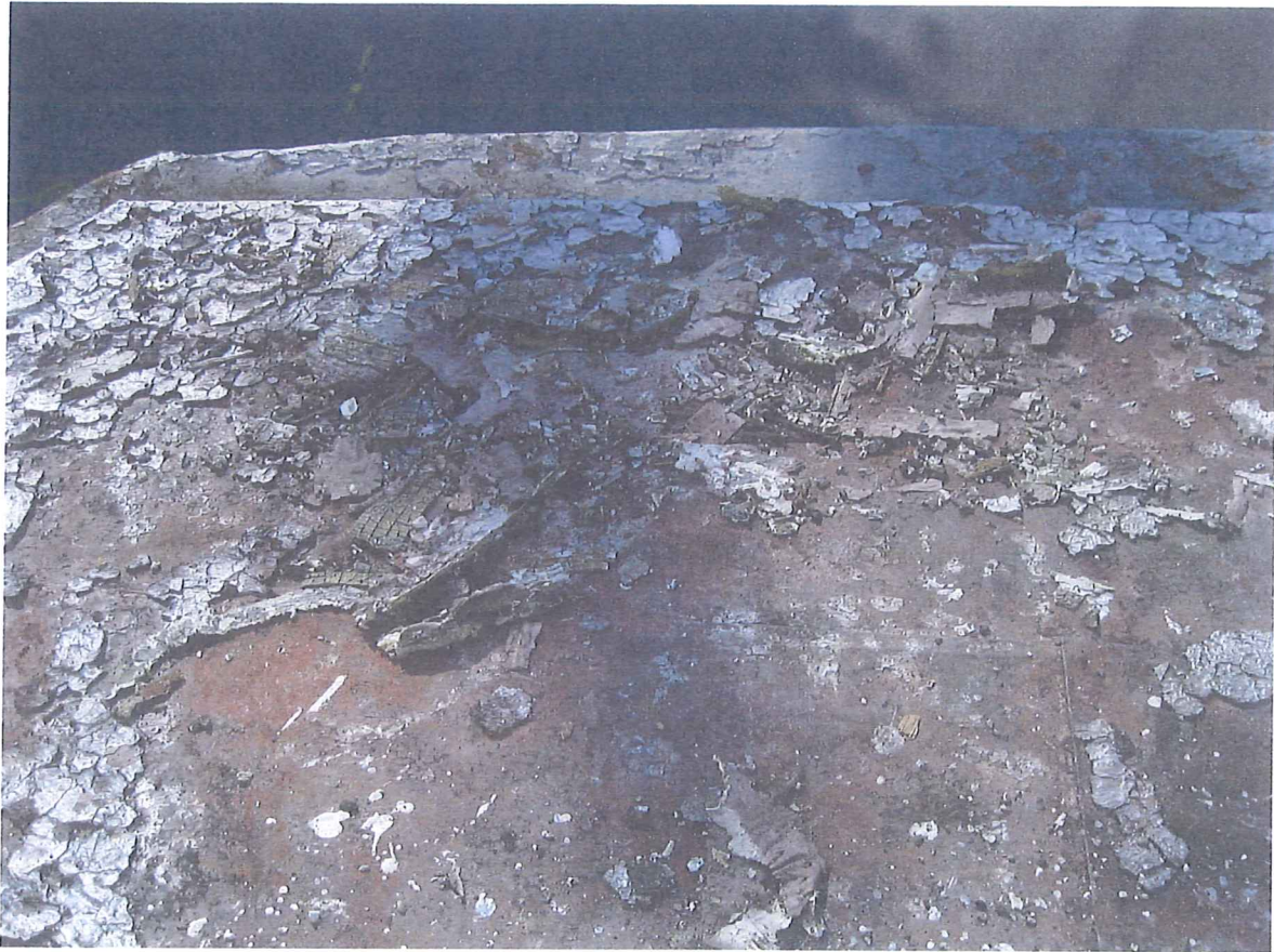
Current state of roof.
