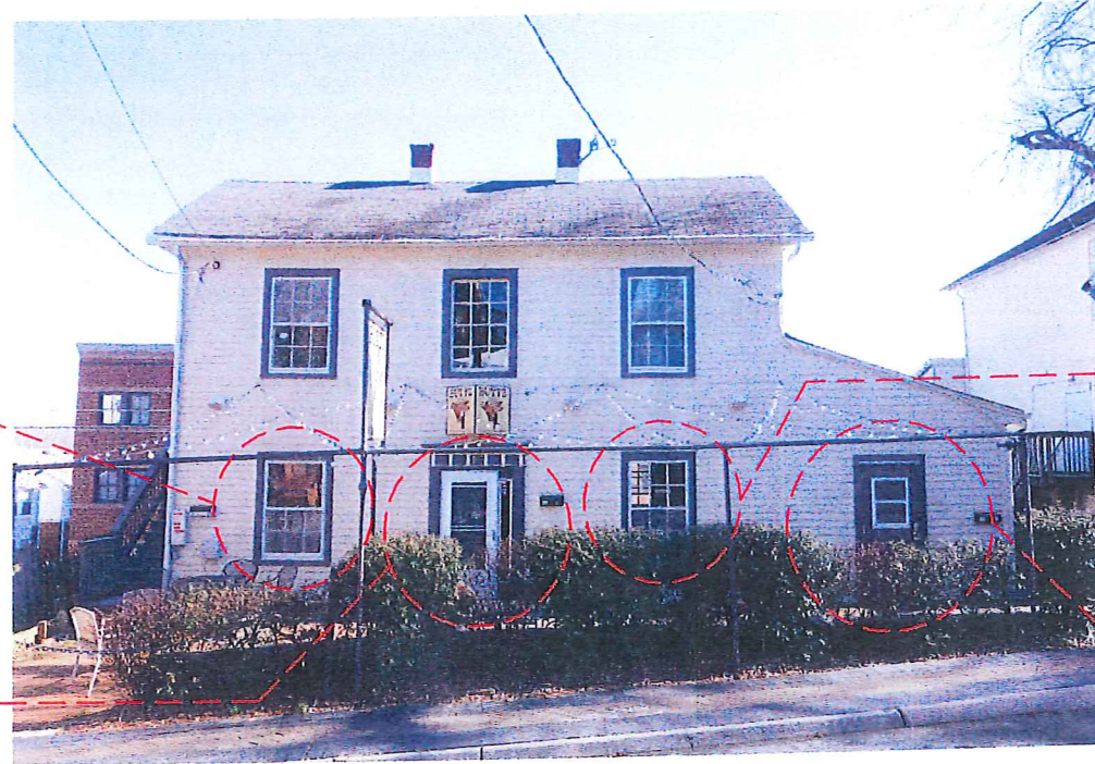
THE UPPER SASH OF THIS WINDOW IS NOT ORIGINAL TO THE BUILDING.
