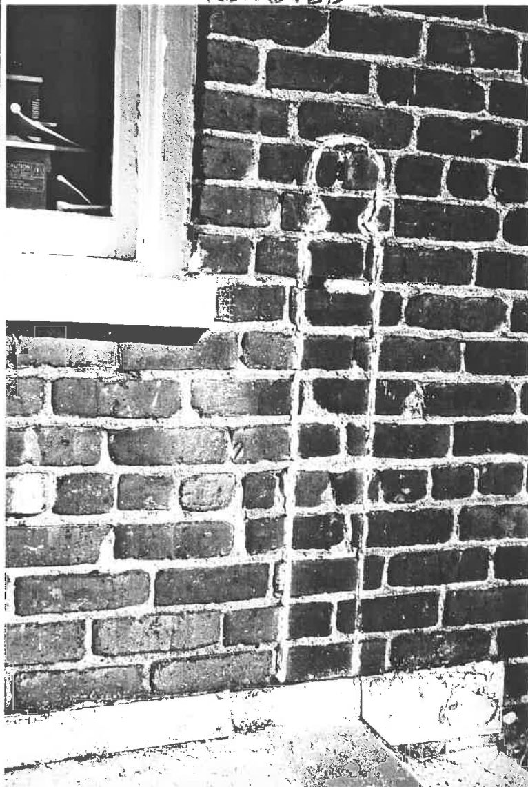
EXISTING BACK PORCH POST OUTLINE WHERE UPPER RAILING WAS REMOVED
