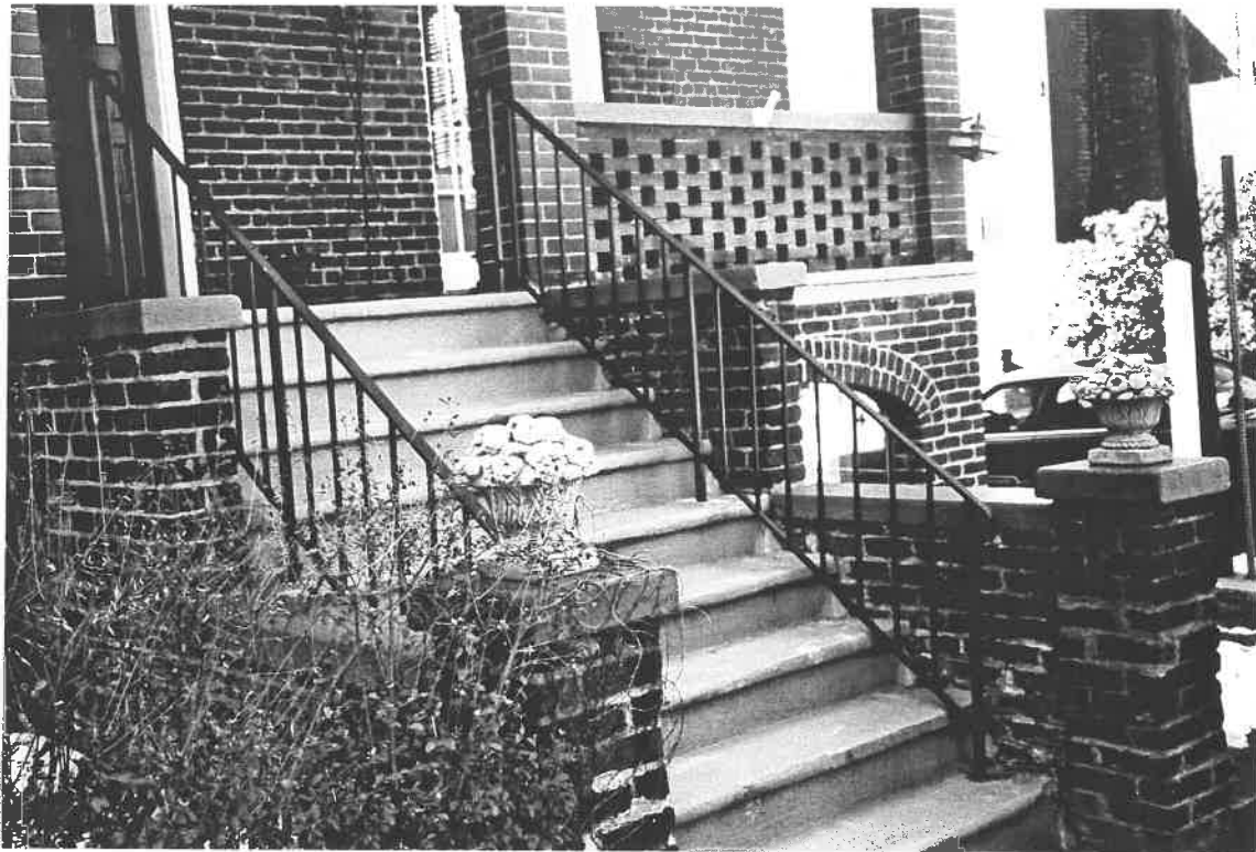
EXISTING STAIR HAND RAILING
