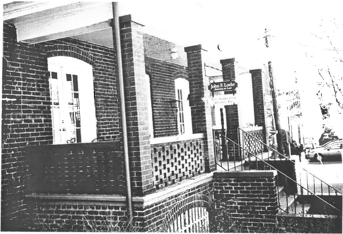
EXISTING FRONT PORCH
