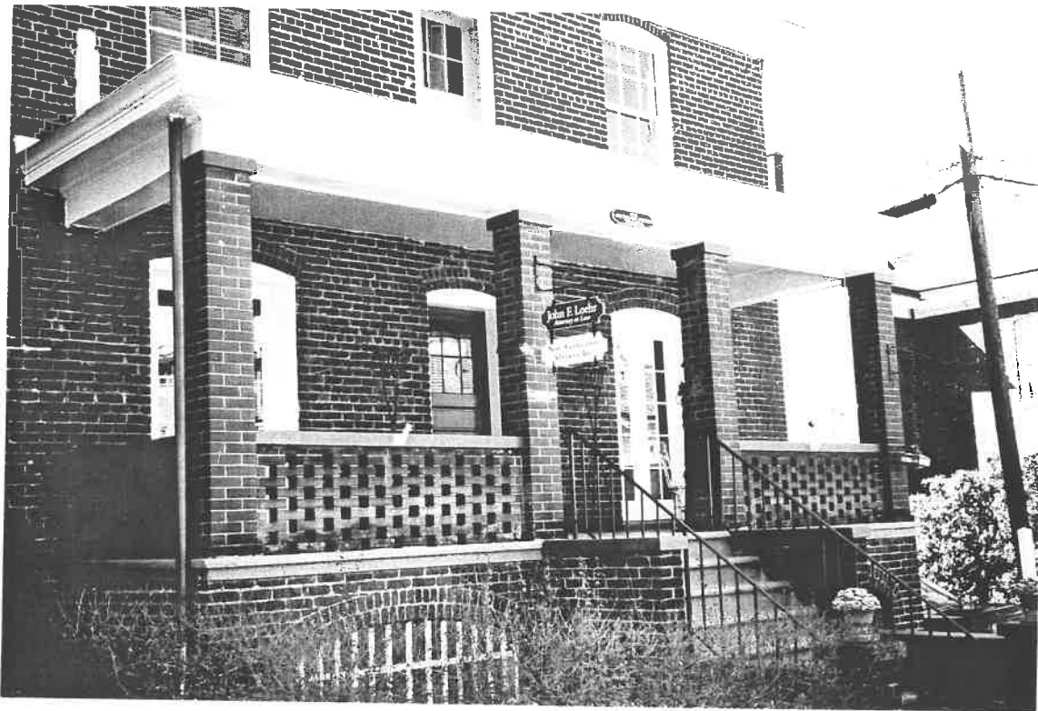
EXISTING FRONT PORCH
