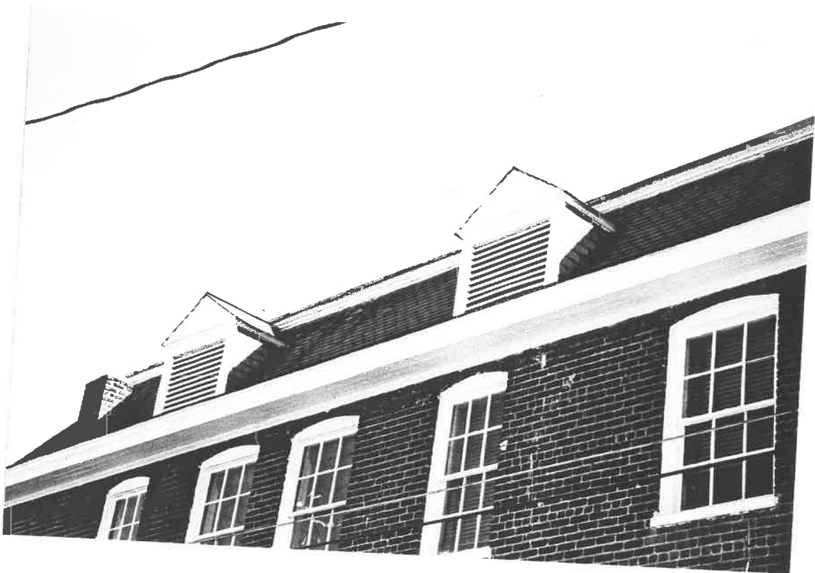
WEST ROOF WITH DORMERS
