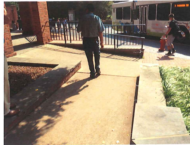
EXISTING CONCRETE RAMP AT BUILDING ENTRANCE
