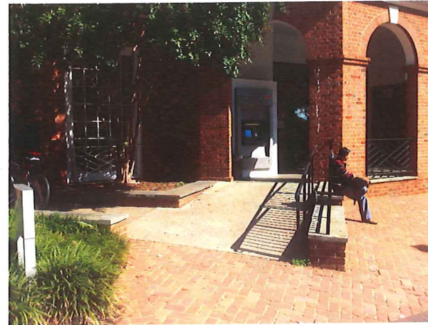
EXISTING BRICK PAVING AND CONCRETE RAMP AT BUILDING ENTRANCE
