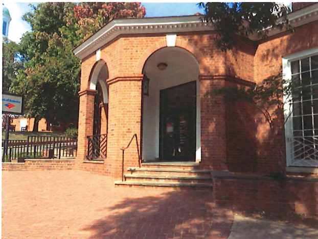
EXISTING BRICK PAVING AND STAIRS
