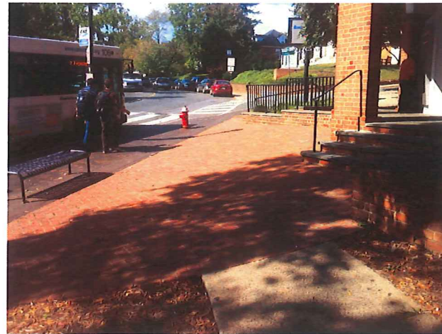
EXISTING BRICK PAVING AT BUILDING ENTRANCE
