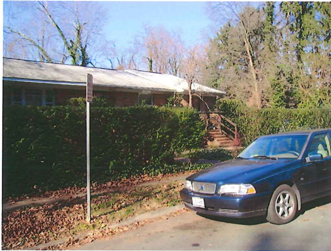
View of existing stoop
