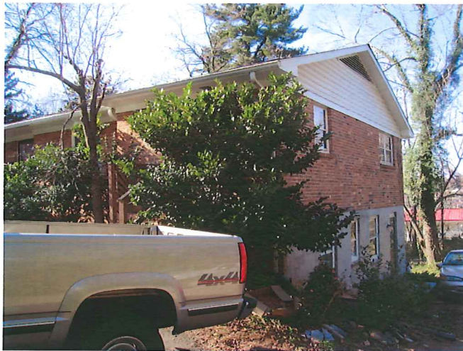
View of proposed deck location
