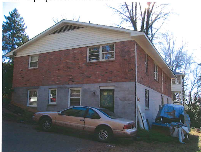
Side and rear view
