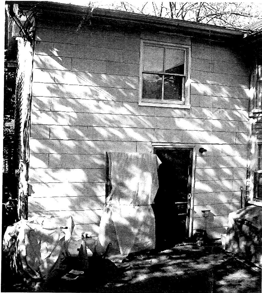
North Elevation (east side)
