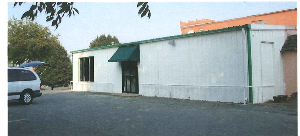
METAL ANNEX & SIDE DRIVE
