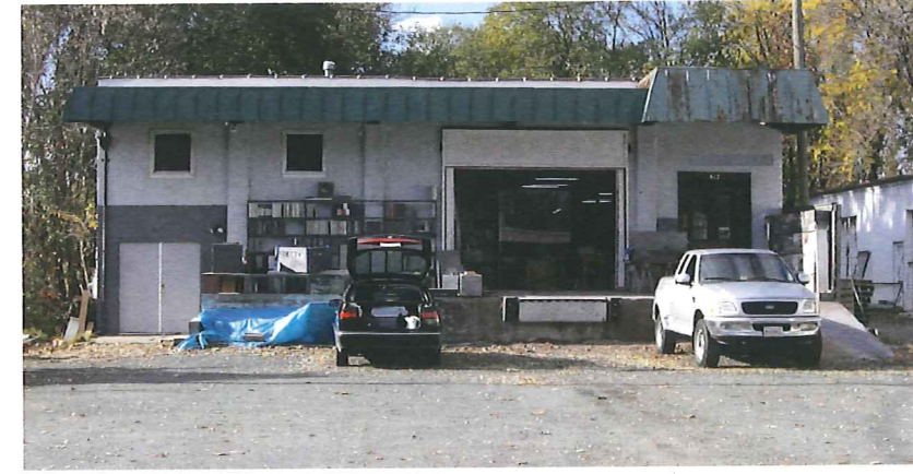
Pretty Hard Concrete
