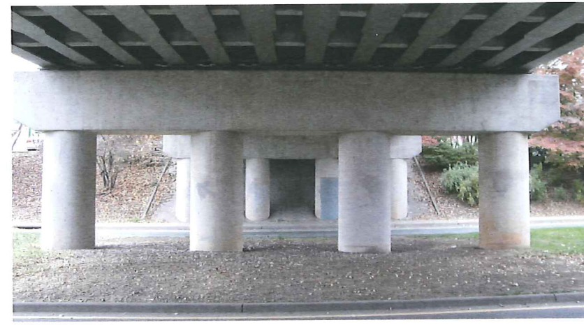
Rail Road Bridge
