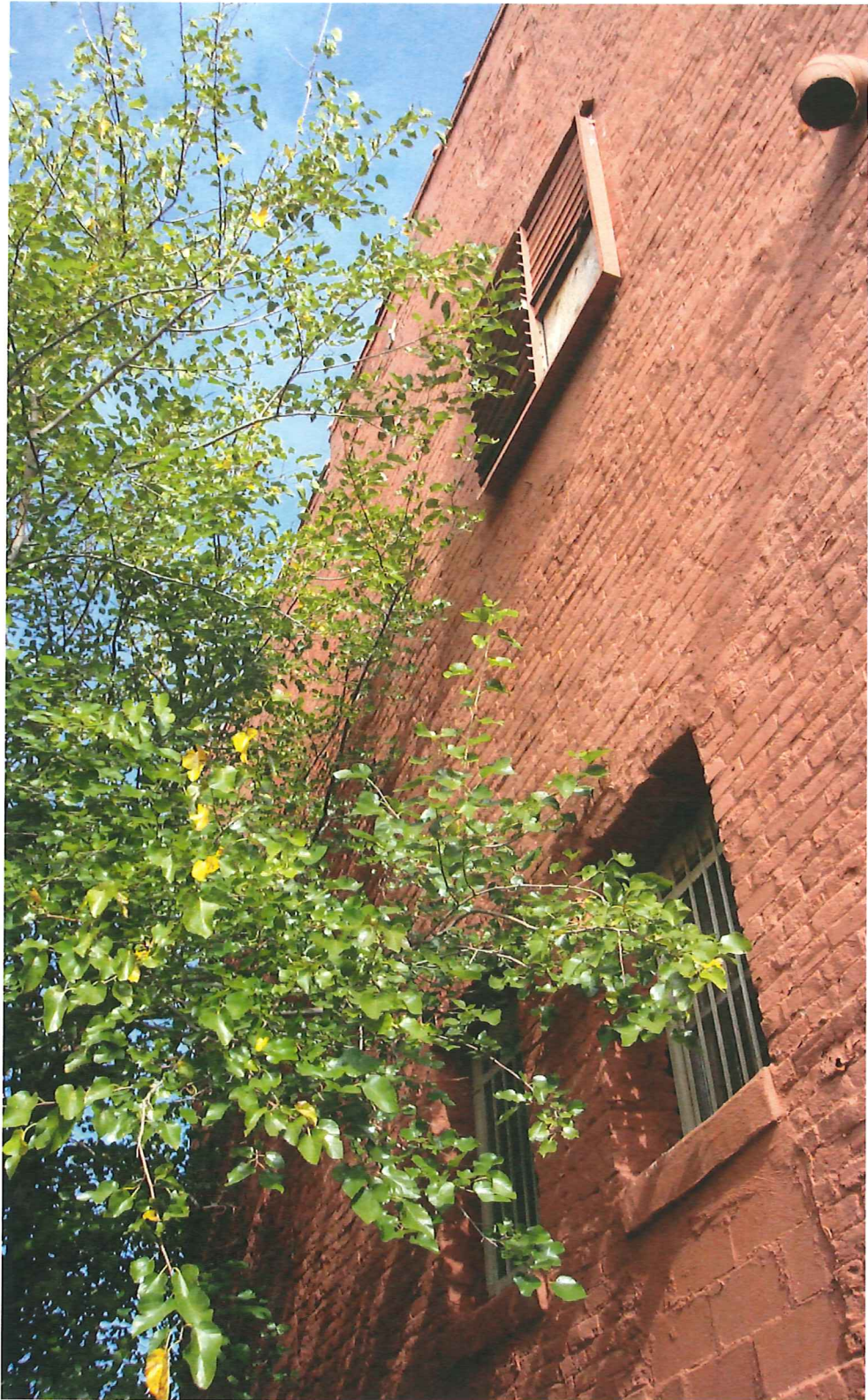
REAR HISTORIC EXTERIOR
