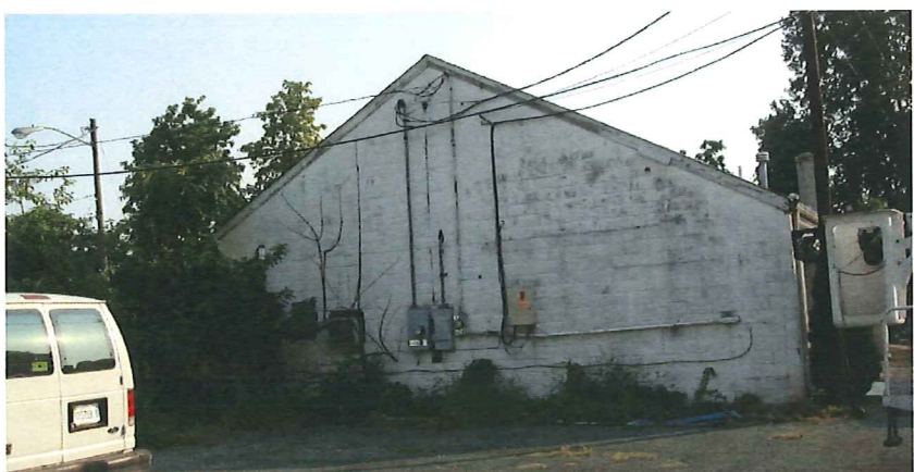
Industrial Building (CMU)
