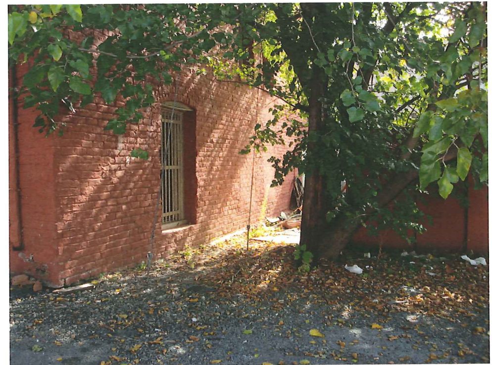
HISTORIC REAR EXTERIOR
