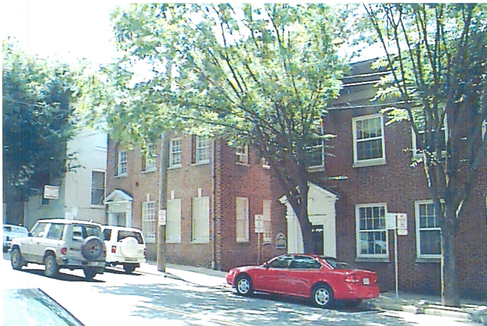
Corner view of 300 and 308 East Market Street
