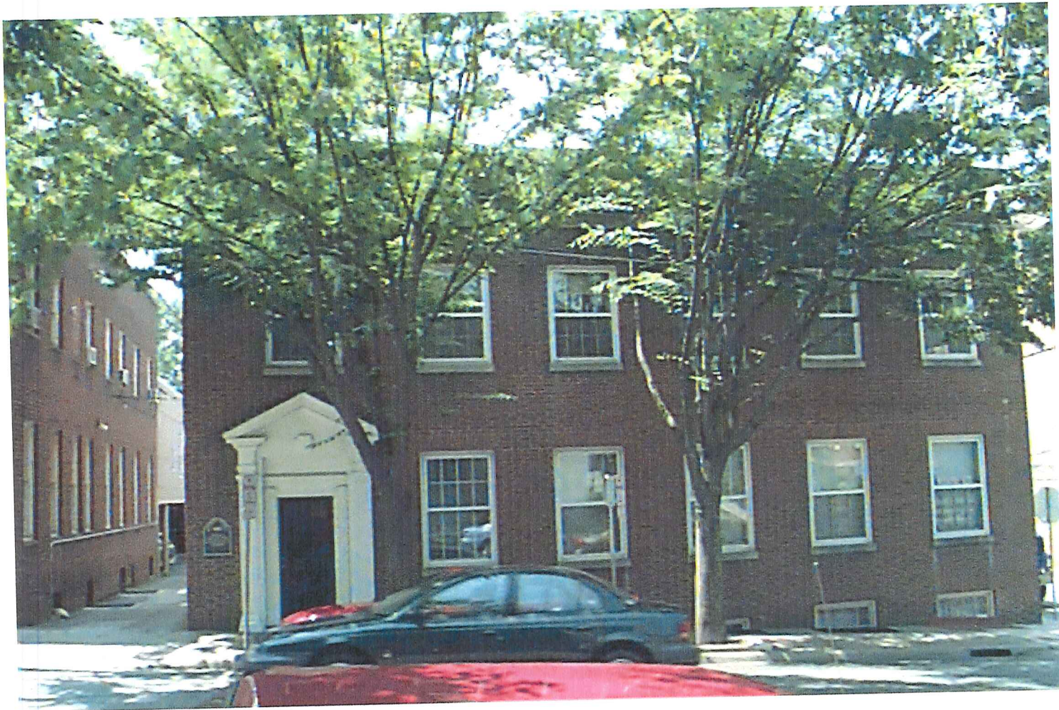
Front view of 300 East Market Street
