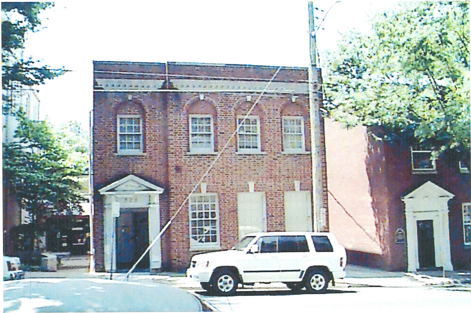
Front view of 308 East Market Street
