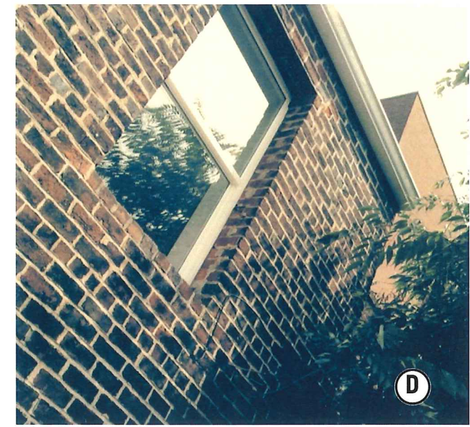
RAW MASONRY JAMBS EXPOSED
