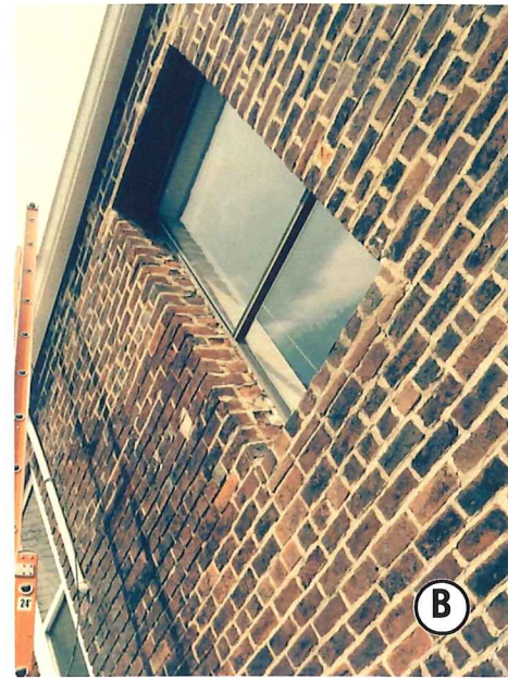
RAW MASONRY JAMBS EXPOSED
