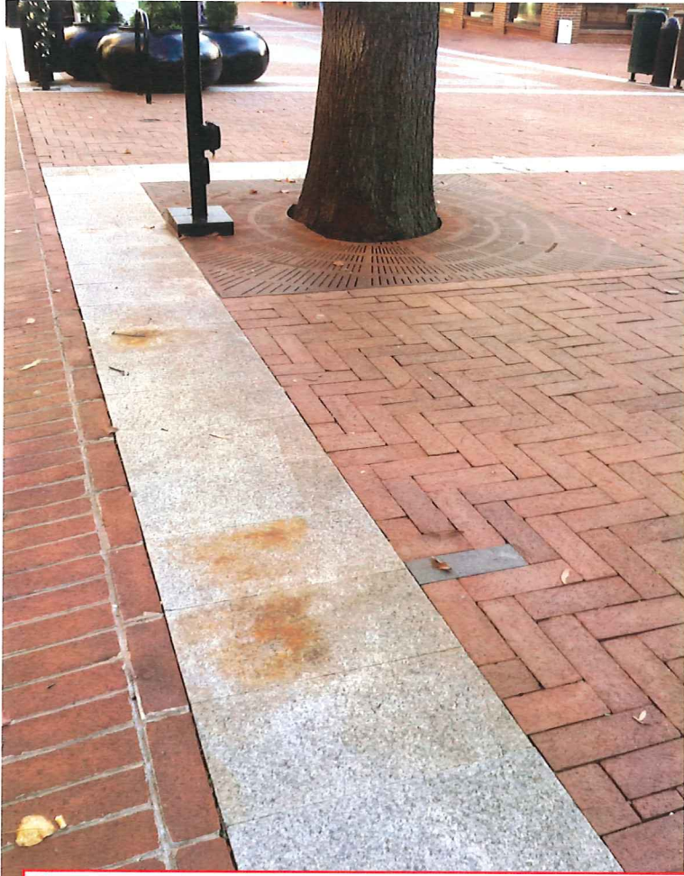
These are photos of the steel grates around the trees on The Downtown Mall. In these Photos we see how difficult it is for the rusting to visually, or otherwise, penetrate onto and effect the brick. One can see the staining from these grates only on the light colored stone. It is the position of Central Place that there will be no visible staining from the proposed Awnings
