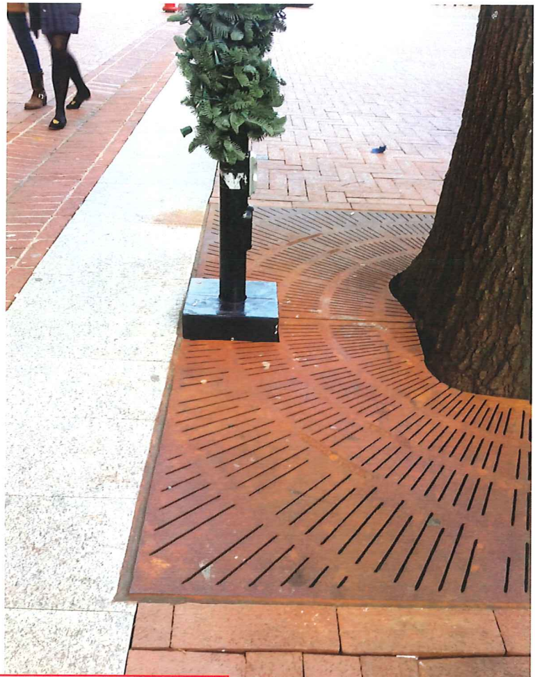
These are photos of the steel grates around the trees on The Downtown Mall. In these Photos we see how difficult it is for the rusting to visually, or otherwise, penetrate onto and effect the brick. One can see the staining from these grates only on the light colored stone. It is the position of Central Place that there will be no visible staining from the proposed Awnings
