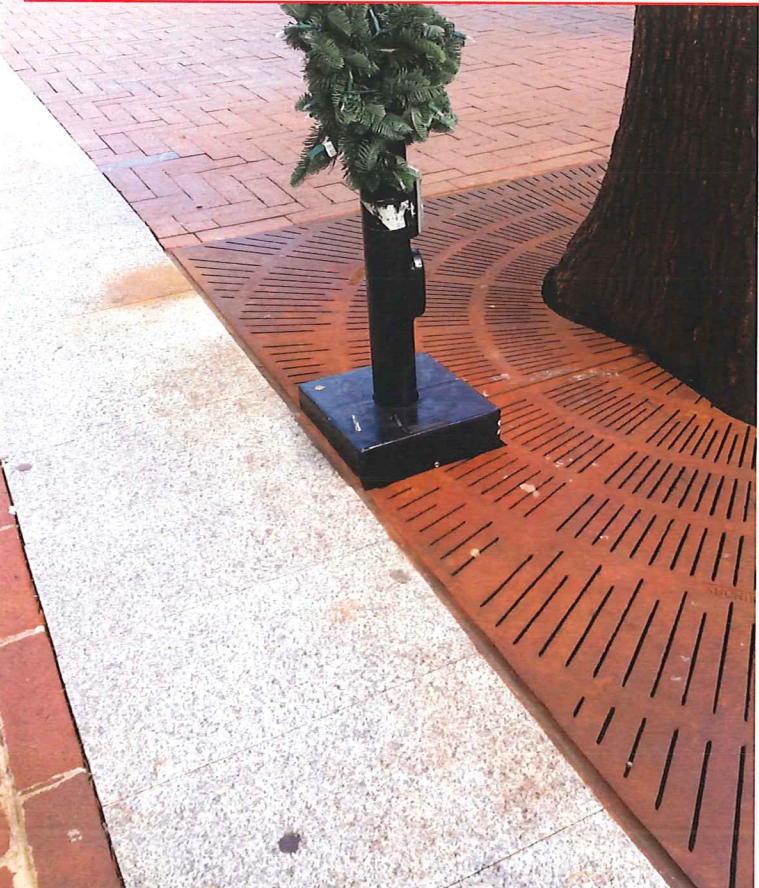
These are photos of the steel grates around the trees on The Downtown Mall. In these Photos we see how difficult it is for the rusting to visually, or otherwise, penetrate onto and effect the brick. One can see the staining from these grates only on the light colored stone. It is the position of Central Place that there will be no visible staining from the proposed Awnings
