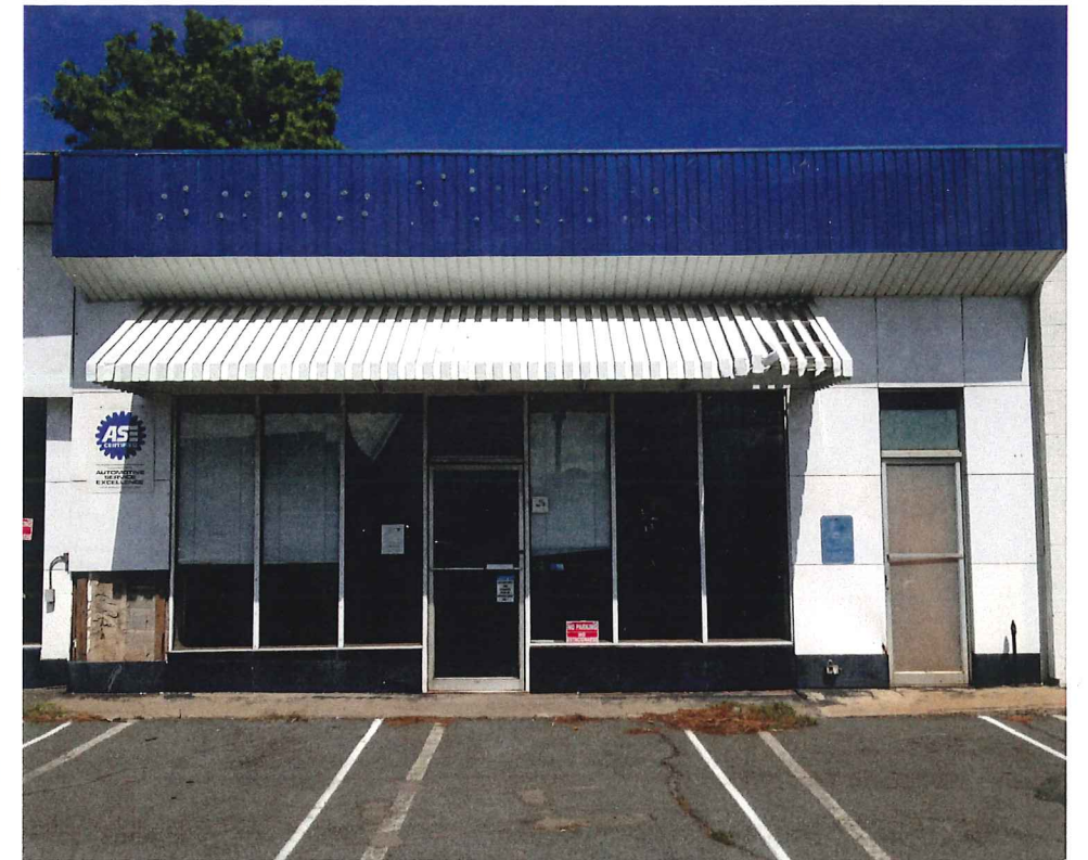
WEST MAIN STREET FACADE
