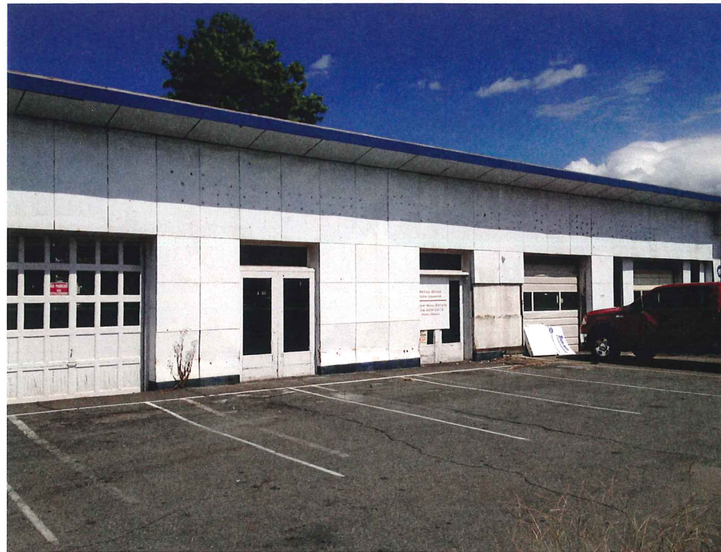
WEST MAIN STREET FACADE
