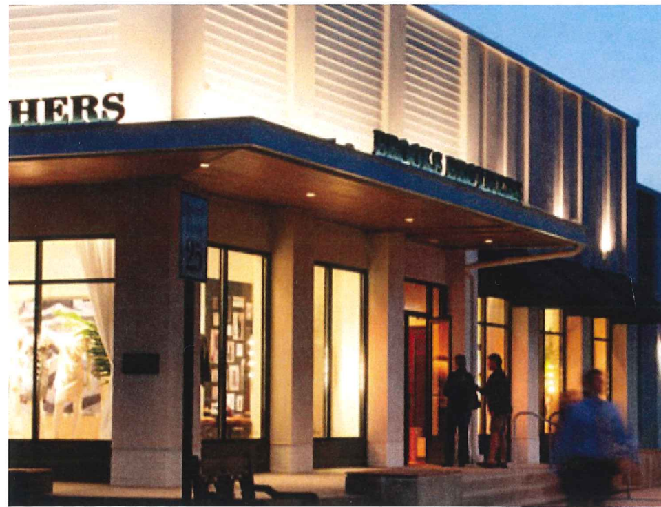
WOOD CANOPY WITH C-CHANNEL STRUCTURE
