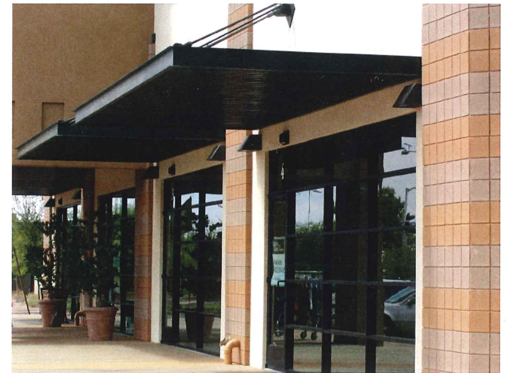
WOOD CANOPY WITH C-CHANNEL STRUCTURE
