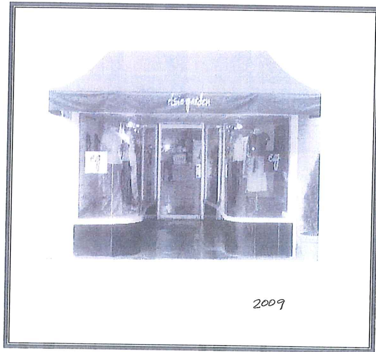
Storefront shows same curved glass with stone base showing window displays for retail goods. Fabric canopy is fixed over façade entry.
