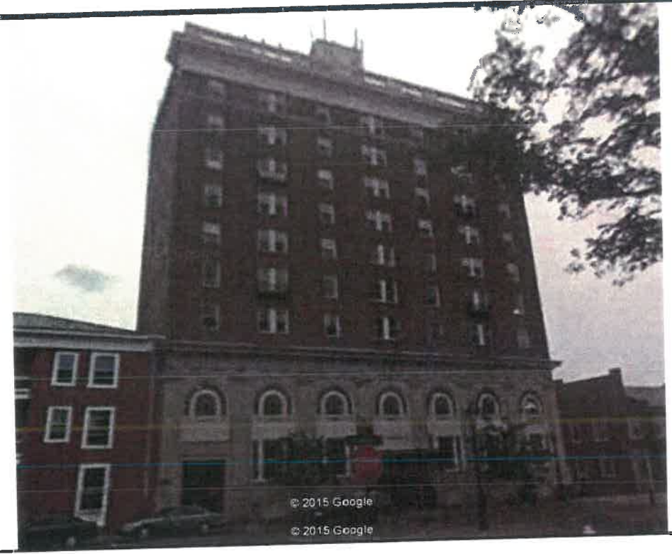
EXISTING BUILDING ELEVATION
