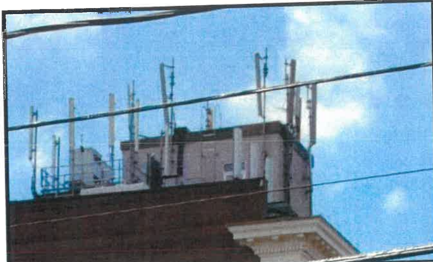
EXISTING ANTENNAS (EAST)
