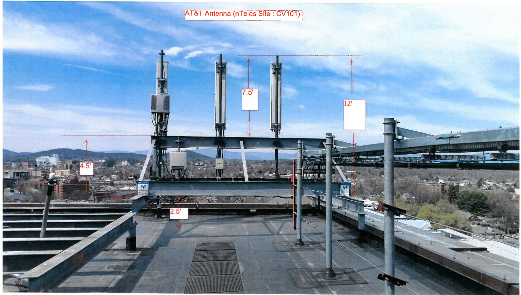
CV 101 (AT&T Antenna Height) NWcorner
