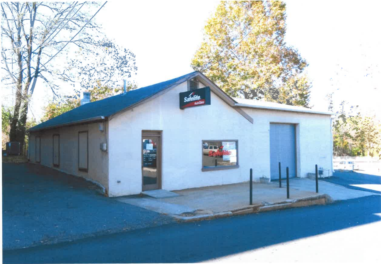
VIEW OF EXISTING BUILDING LOOKING NORTHWEST FROM 8TH ST. NW
