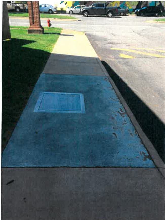
Friendship Court – Drive Entrance off of Monticello Ave (retrofit installation in 2013)
