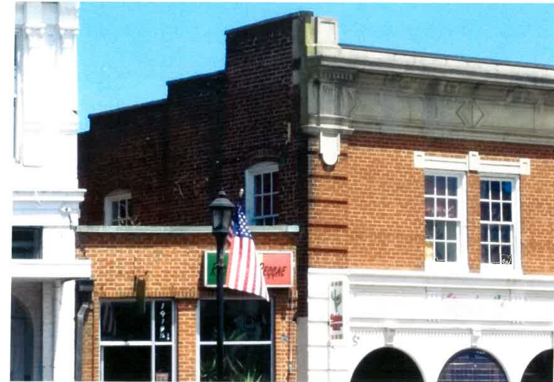
View of west side of building
