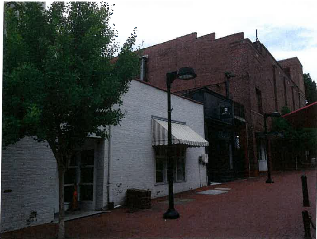
Buildings on Contiguous properties – Third Street NE
