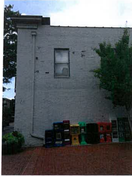
Façade – Third Street NE
