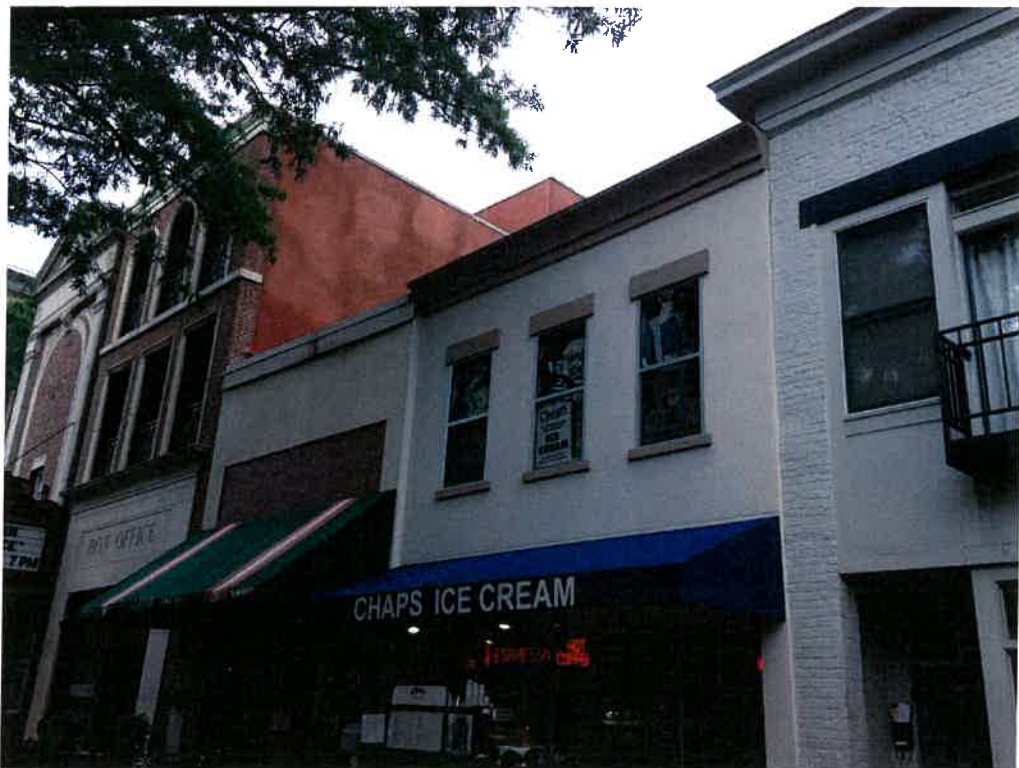
Buildings on Contiguous properties – East Main Street
