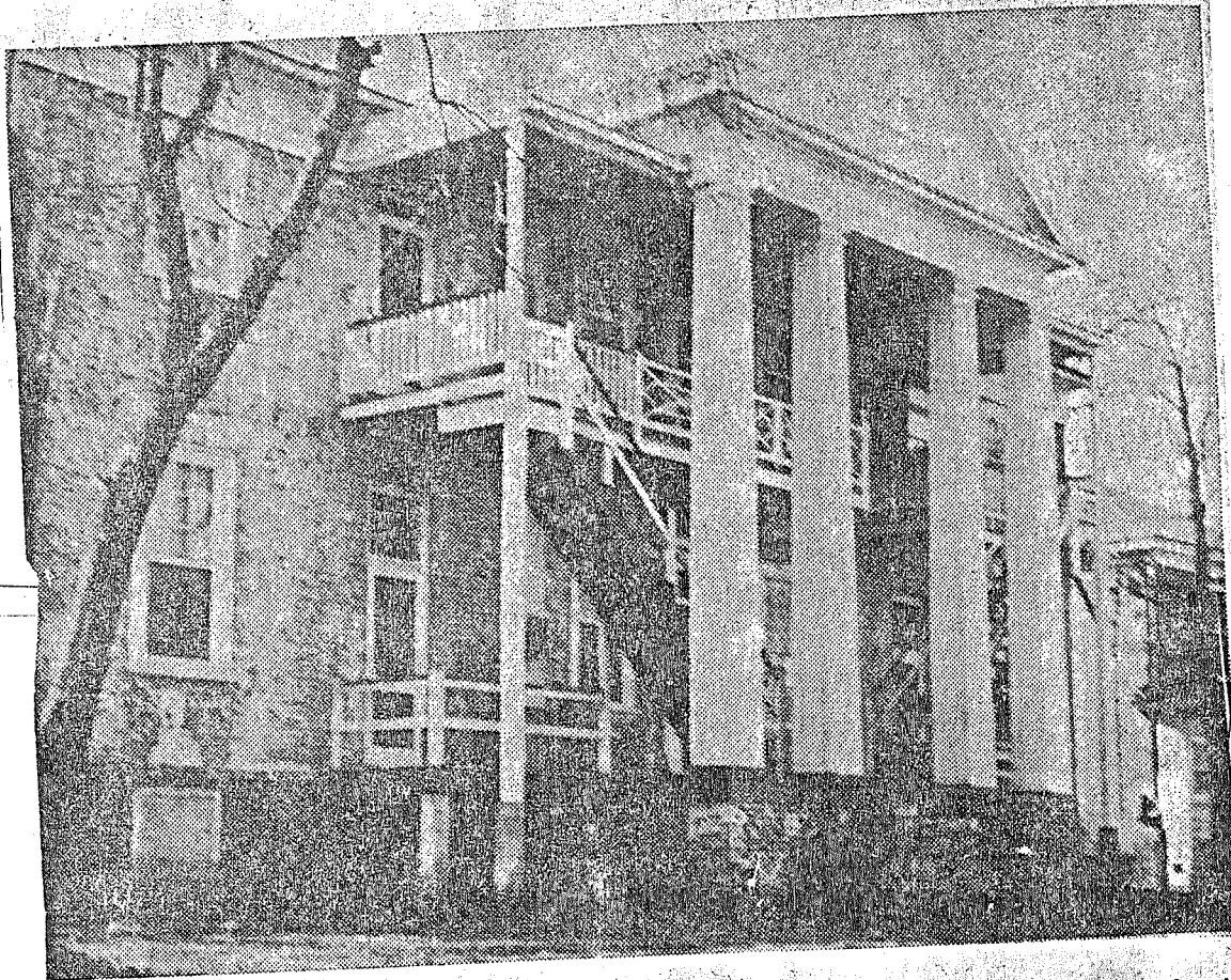
FORMERLY CALLED "BELLE-MONT," this is the original part of the old Belmont Stock Farm which gave its name to the part of Charlottesville which grew up on its property. Now an apartment building, this old part which was the front entrance, is now the rear of the house. John Carr, John Winn and Slaughter Ficklin all owned the home.
