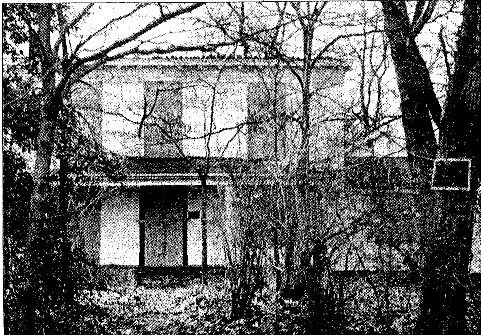
Progress photo by Matt Gentry
