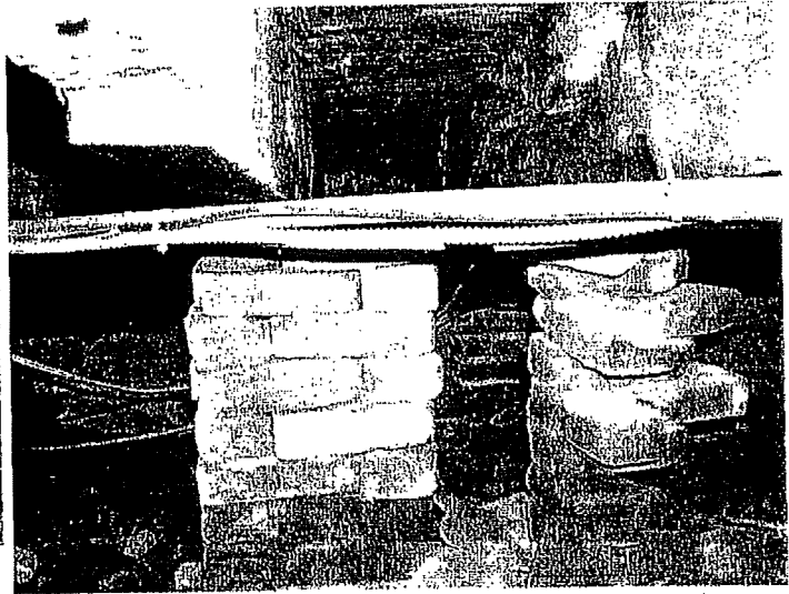
Inadequate Brick Piers under High Addition
