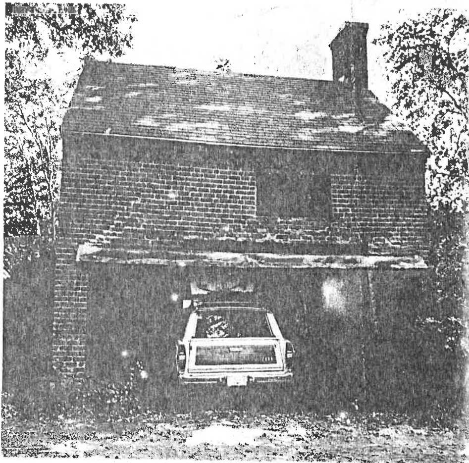
MODEST KITCHEN BUILDING NOW SERVES AS GARAGE Not Fine Old Brickwork in Building's Cornice
