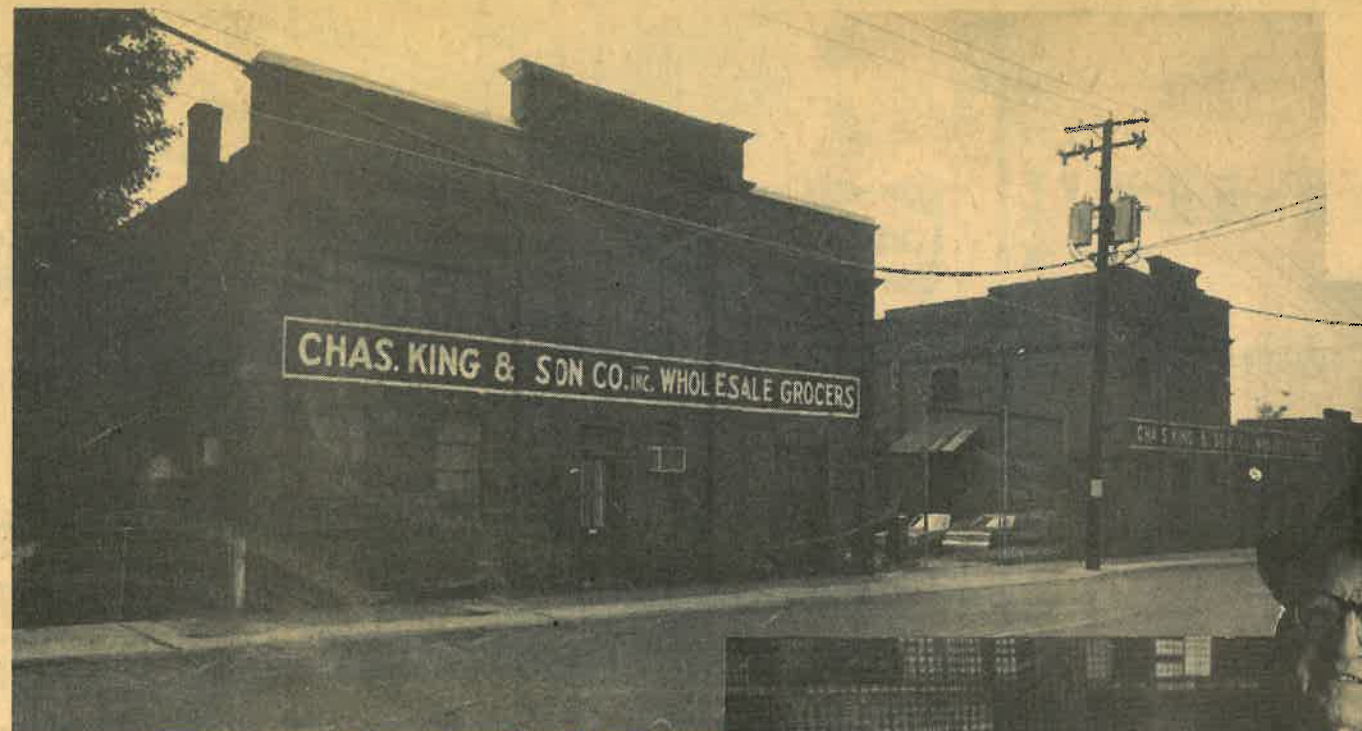
Progress Photo by John Atkins
