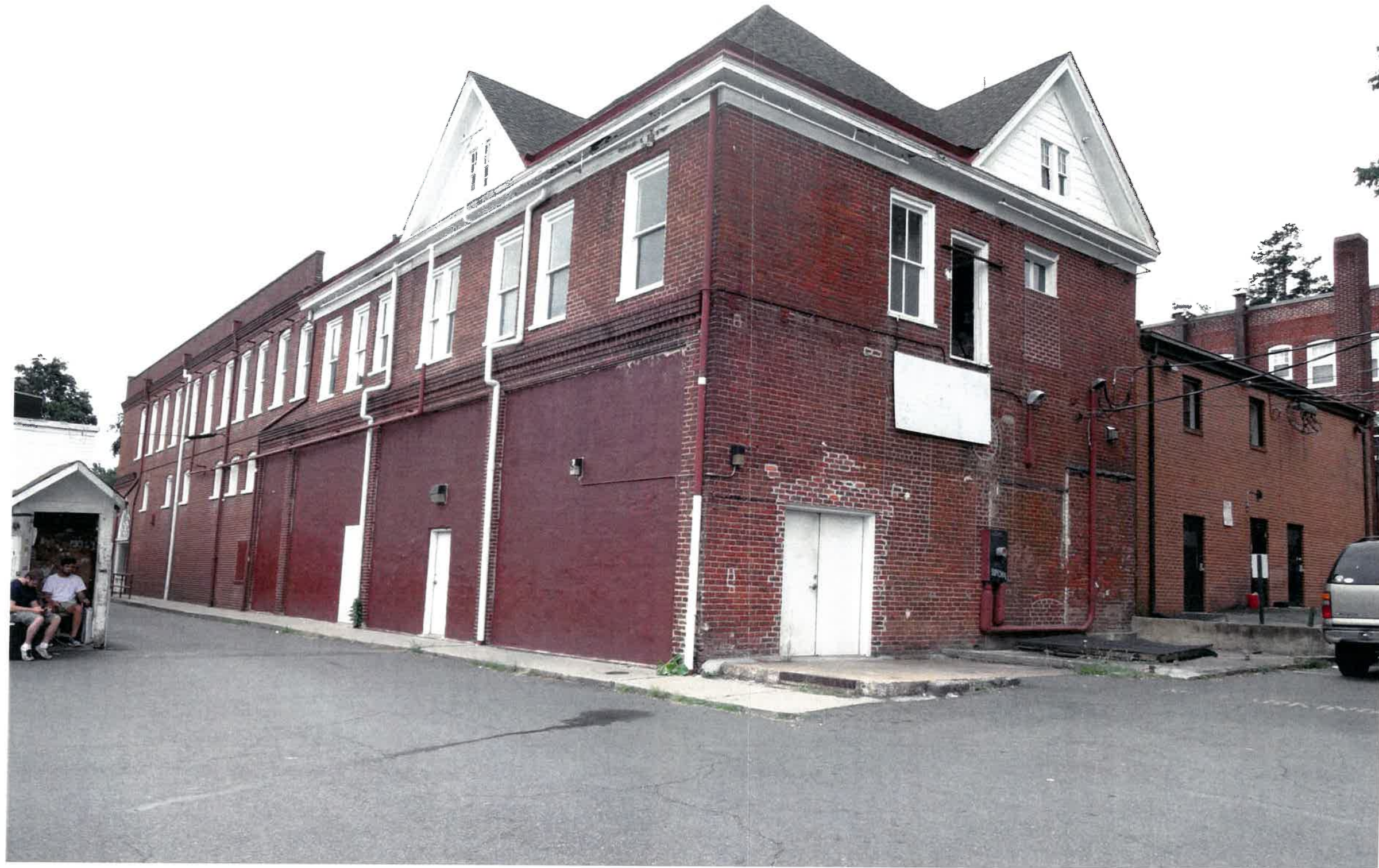
Existing View From North East Corner
