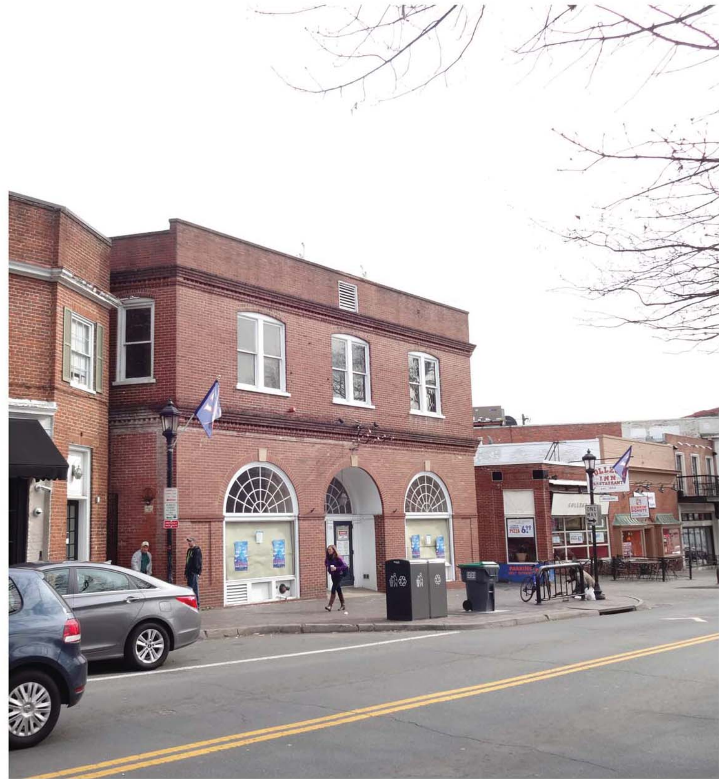
FRONT VIEW FACING EAST
