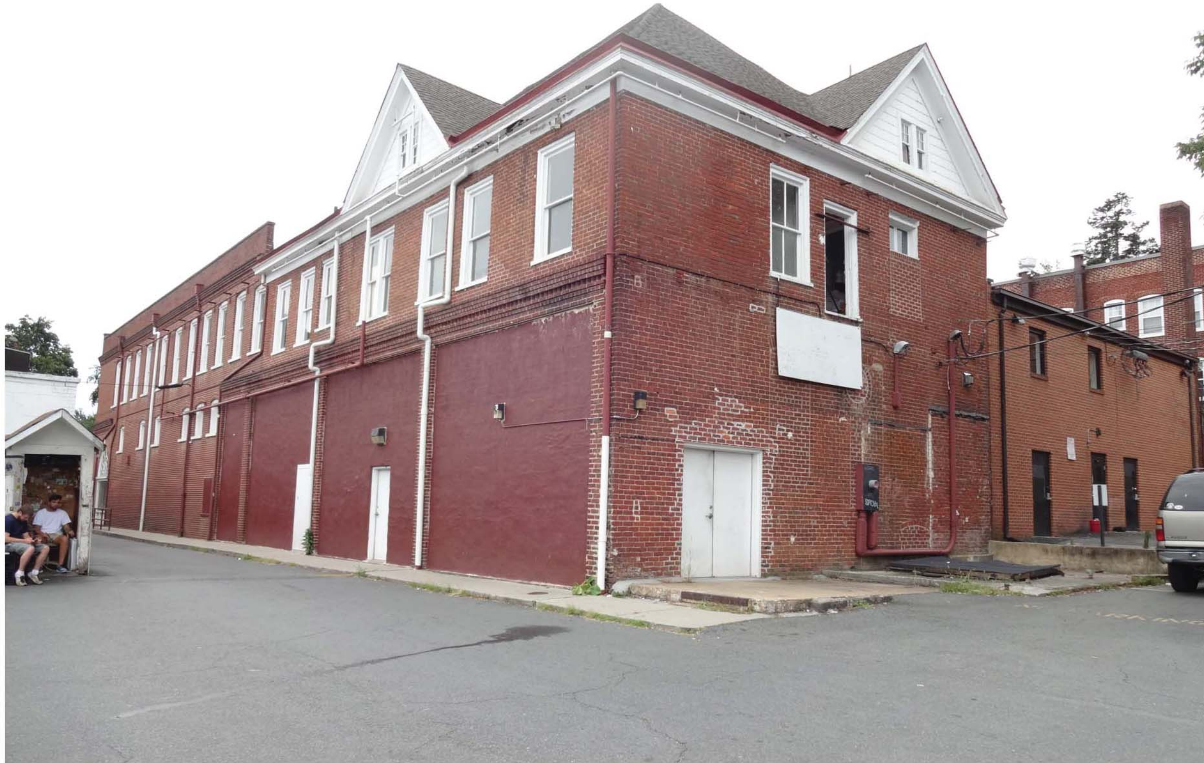
EXISTING VIEW FROM NORTH-EAST CORNER
