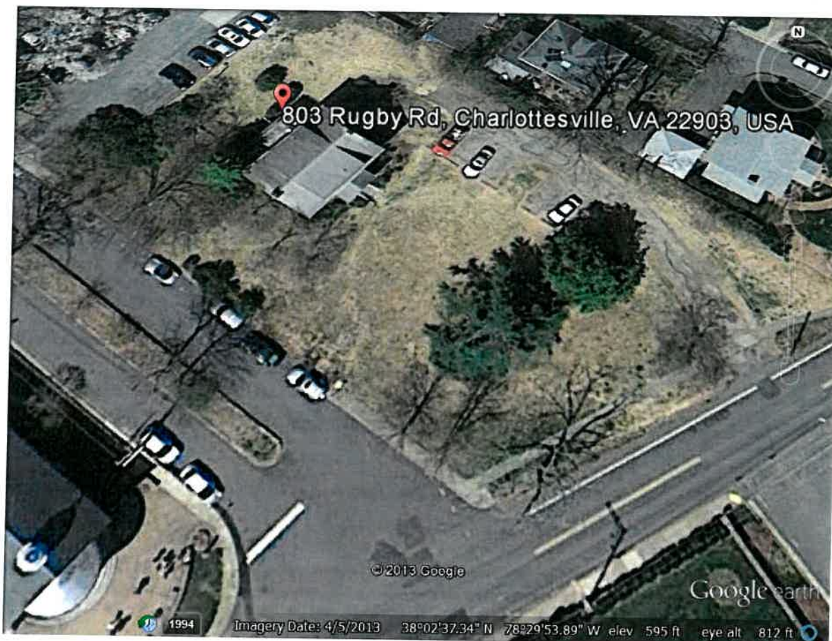
Aerial View of 803 Rugby Road [Source: screen shot from Google Earth]
