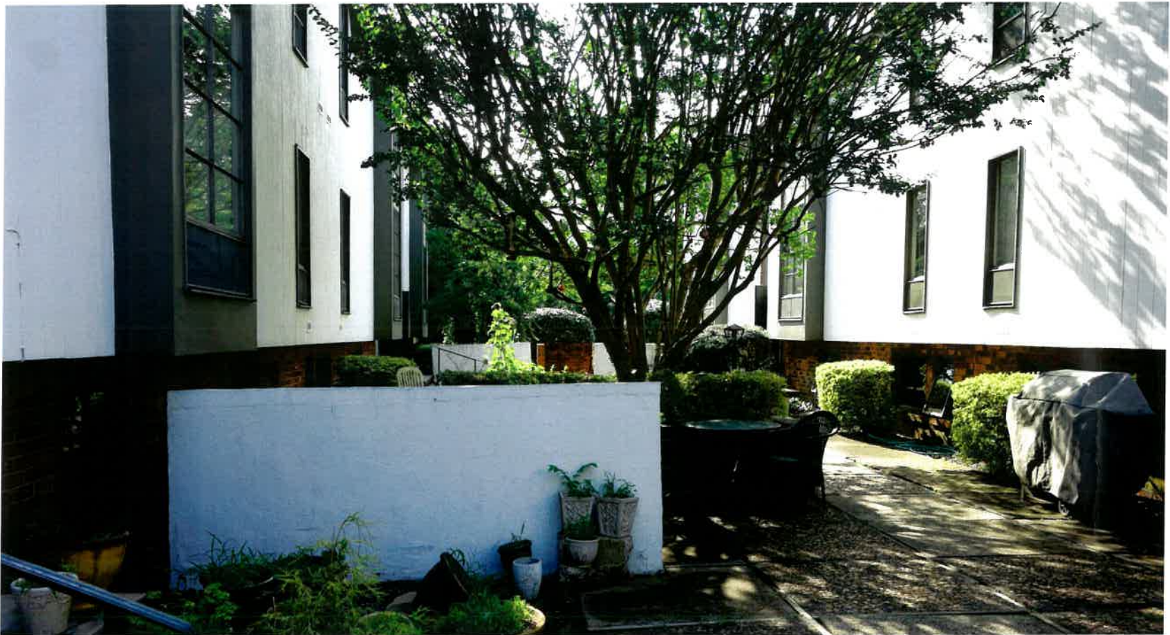
Existing Central Courtyard with site walls and raised planter
