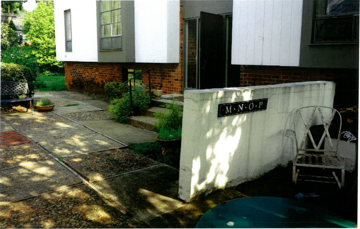
Existing paving a mix of concrete, exposed aggregate and brick
