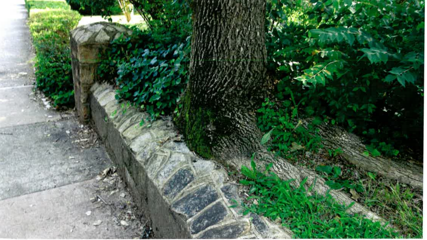
Existing 12" White ash tree to be removed over historic stone wall
