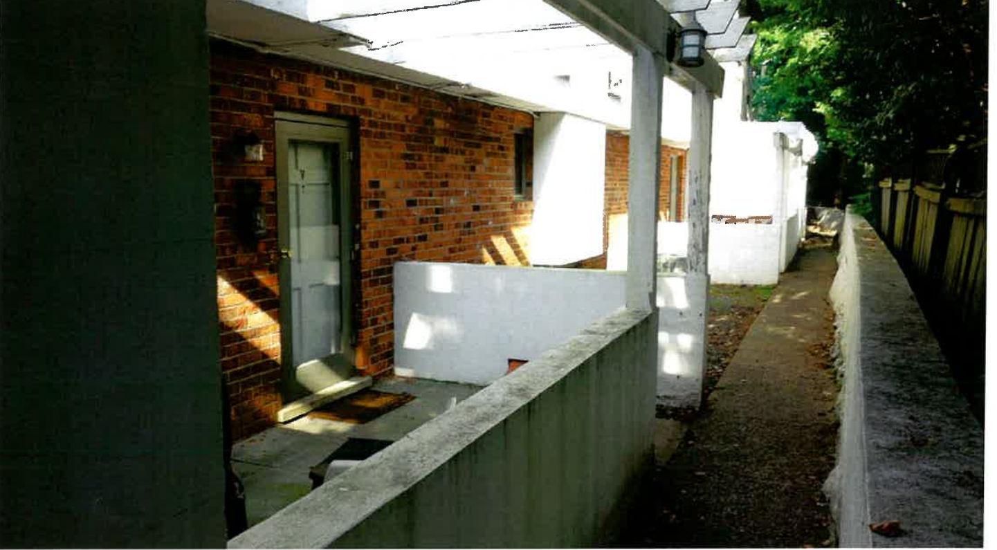
North courtyards facing site wall and back of neighbor's fence
