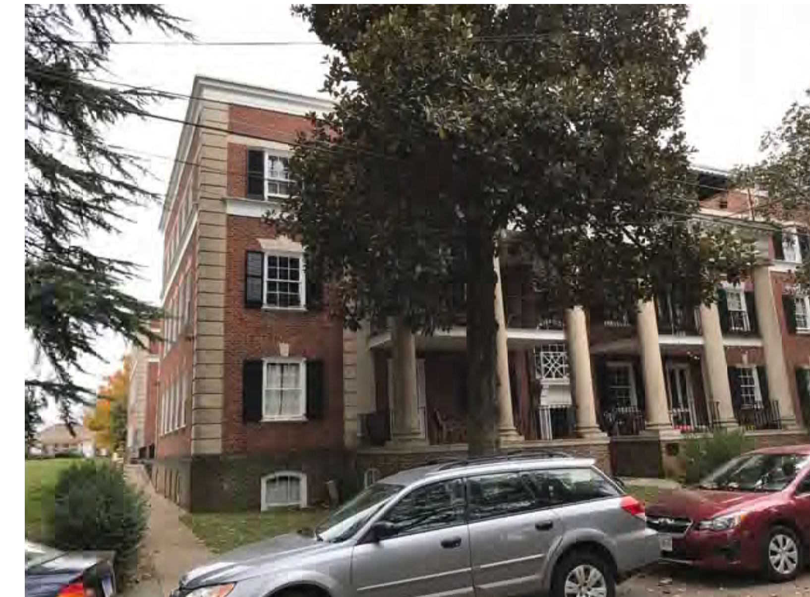
EXISTING CONDITIONS - NORTHWEST CORNER
