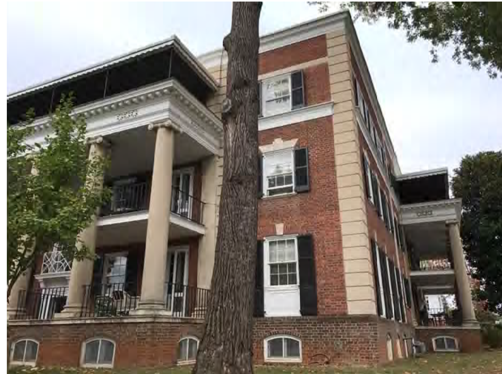
EXISTING CONDITIONS - SOUTHEAST CORNER
