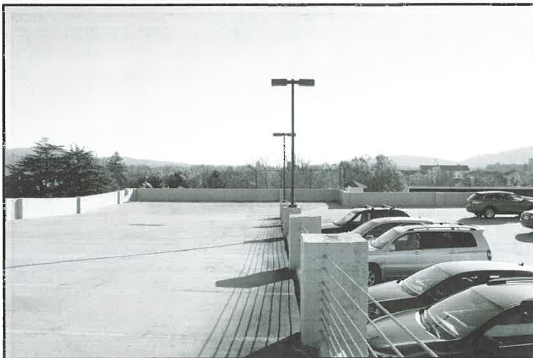
Figure 11. Views from Roof Level 301 15 th Street NW Collocation Site (UVA MC N009), Charlottesville, Virginia, Looking East.
