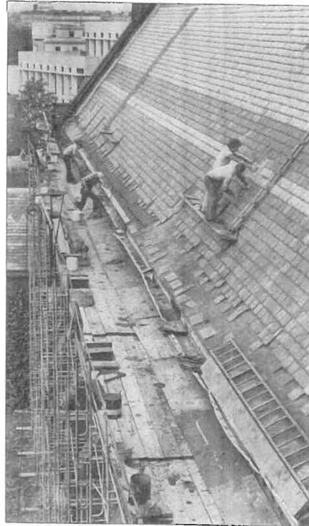
Workmen are in the process of removing deteriorated roofing slates and replacing them with new matching slates.
