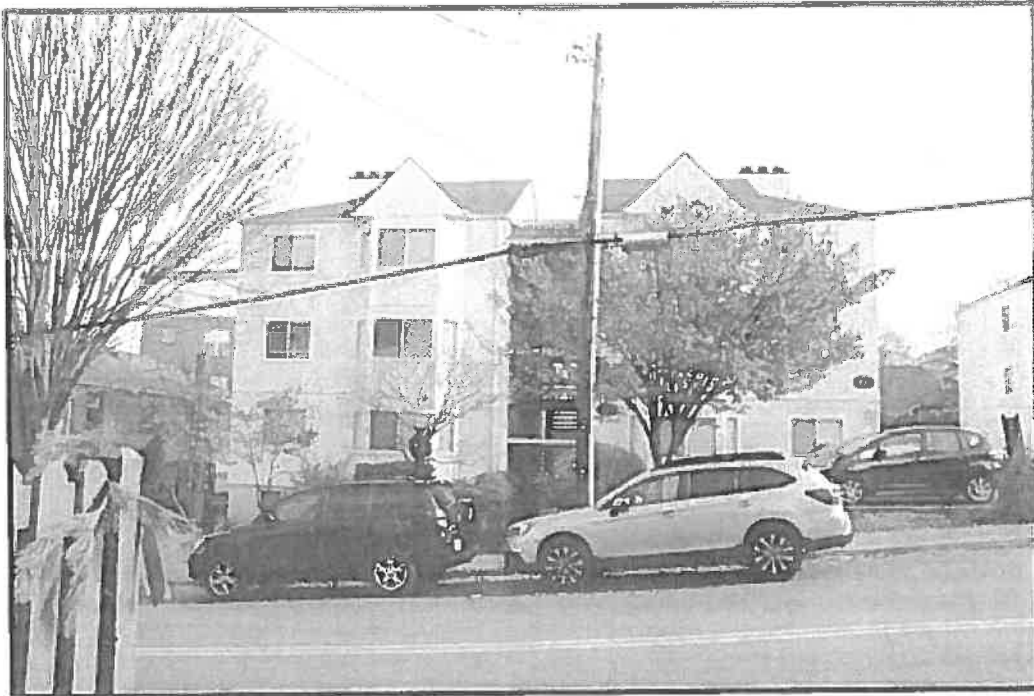
Photo 27. View of Modern Apartment Building, Former Location of McConnell-Neve House (VDHR #104-0397), Looking Southeast (Resource as Plotted in VCRIS Appears to have been Demolished).
