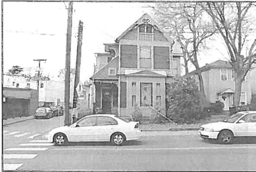
Photo 23. View of King-Runkle House (VDHR #104-0248), Looking West.
