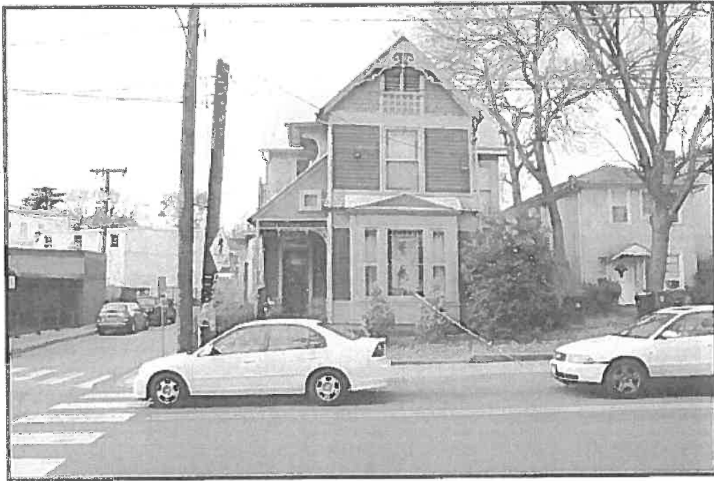
Photo 23. View of King-Runkle House (VDHR #104-0248), Looking West.
