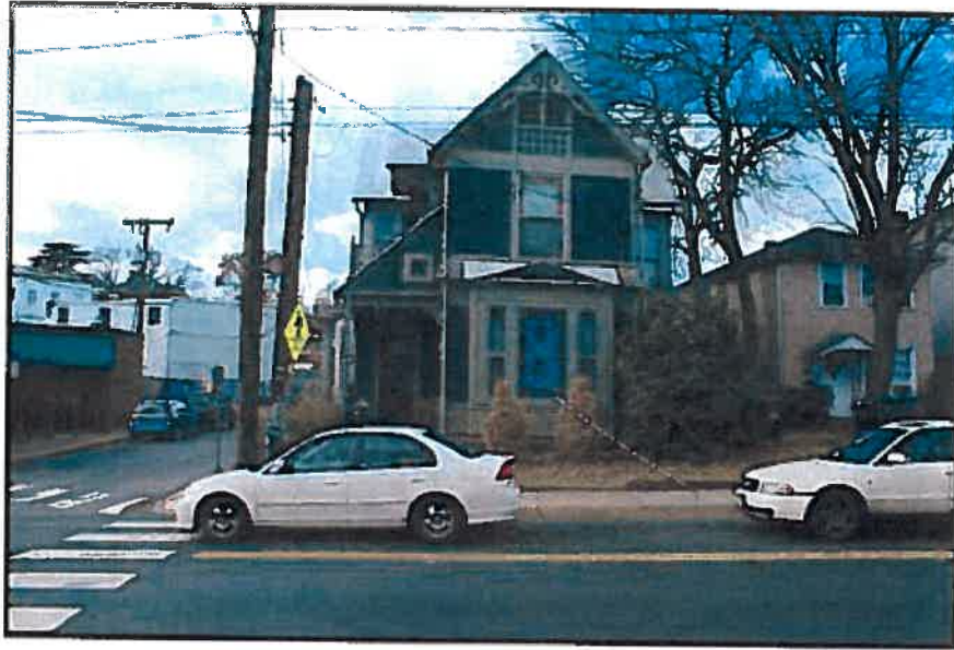
Photo 23. View of King-Runkle House (VDHR #104-0248), Looking West.
