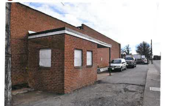
6 10TH STREET NW STRUCTURE
