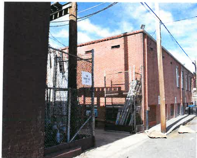
1 DAIRY BUILDING CORNER TO REMAIN
