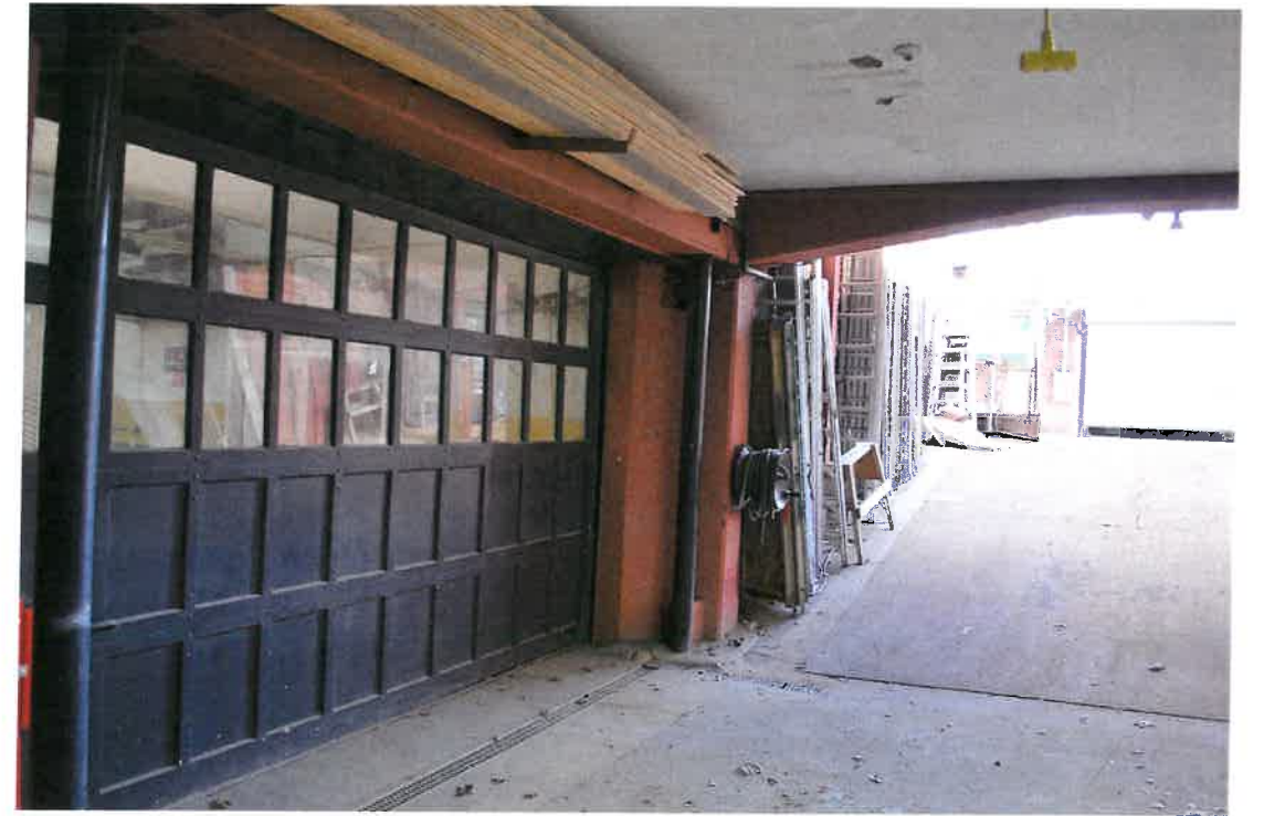
1 VIEW OF REAR WALL FROM LOADING AREA
