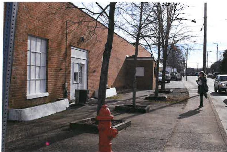
1 WEST ELEVATION LOOKING SOUTH WITH HISTORIC WINDOW
