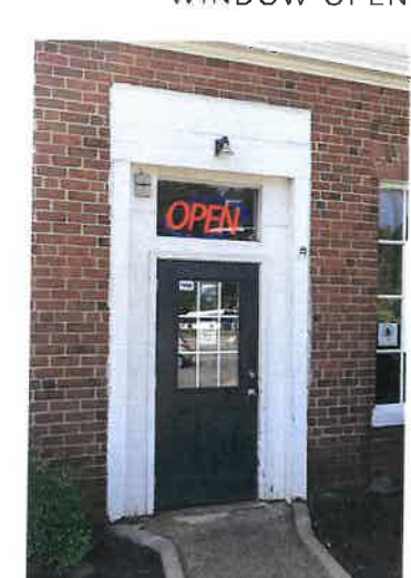
12 ENTRY IN HISTORIC WINDOW OPENING
