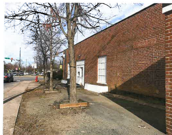
1 WEST ELEVATION LOOKING NORTH NON HISTORIC OPENING TO BE REMOVED, AND HISTORIC WINDOW TO BE RESTORED
