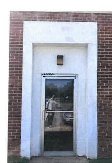
11 ENTRY IN HISTORIC WINDOW OPENING
