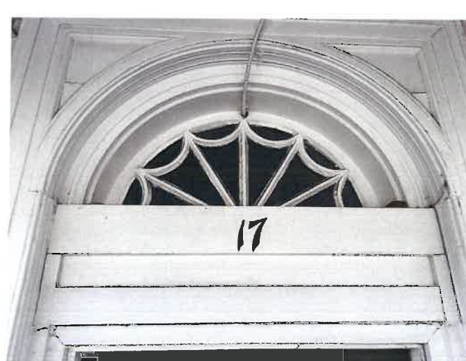
HISTORIC MAIN ENTRANCE FAN WINDOW TO BE RESTORED
