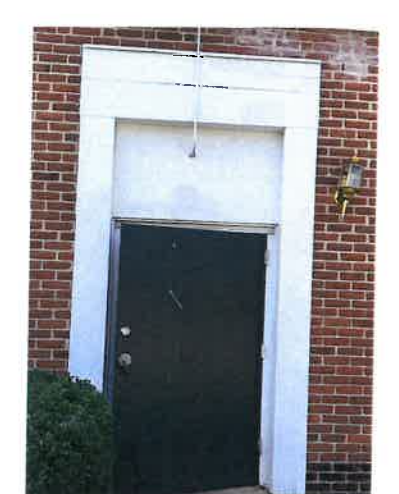
7 ENTRY IN HISTORIC WINDOW OPENING
