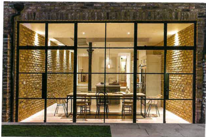
STEEL INDUSTRIAL WINDOWS AT NEW WINDOW LOCATIONS
