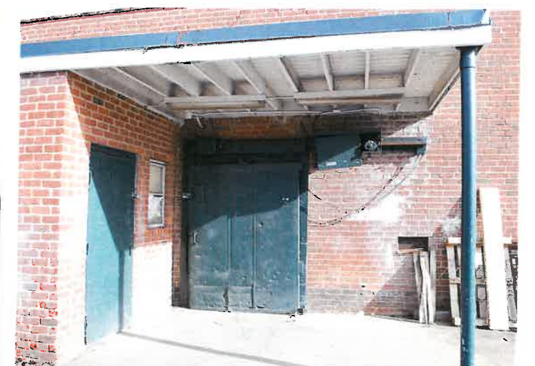
2 INTERIOR OF LOADING BAY ADDITION
