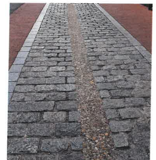
WOOD STREET PAVING
