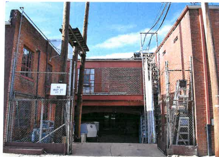
2 AREAWAY TO BE REMOVED, DAIRY CORNER TO REMAIN (RIGHT SIDE)
