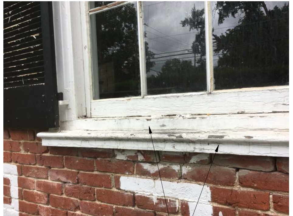
cracking, dents, dry-rot, water damage at sills and sashes - typical
