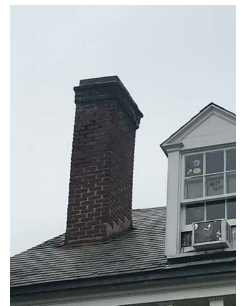
4. Front elevation - 3rd floor window
