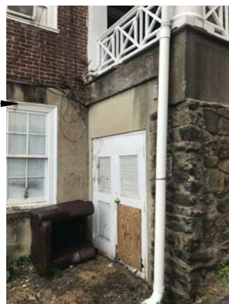
7. South elevation (under porch)
