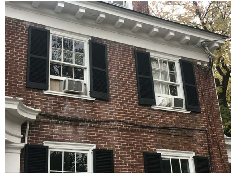
3. Front elevation - 1 & 2nd floor windows
