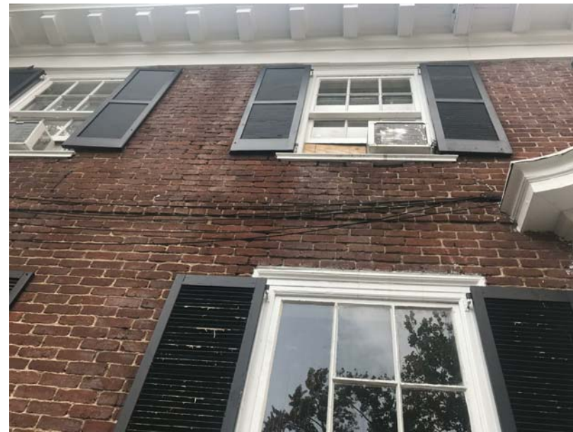
2. Front elevation - 1 & 2nd floor windows
