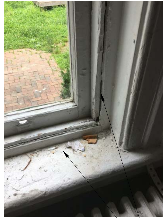
cracking, dents, dry-rot, water damage at interior sills and sashes - typical
