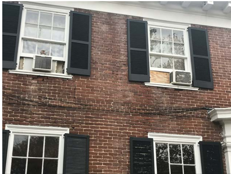
1. Front elevation - 1 & 2nd floor windows
