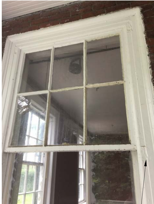
damaged exterior trim
