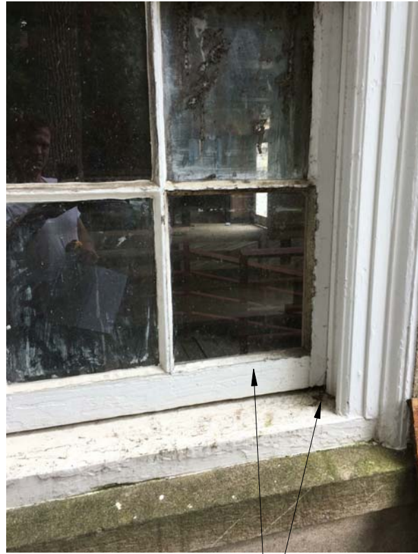
water damage and wood rot
