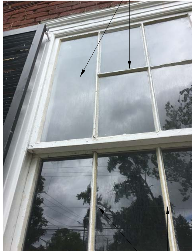
overworked muntins due to repeated reglazing
