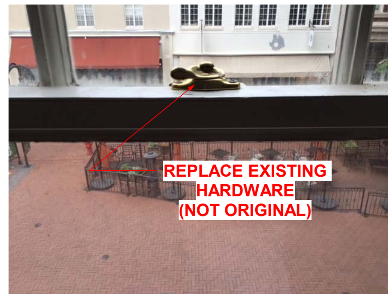
WARPED UPPER SASH TO BE REPLACED
