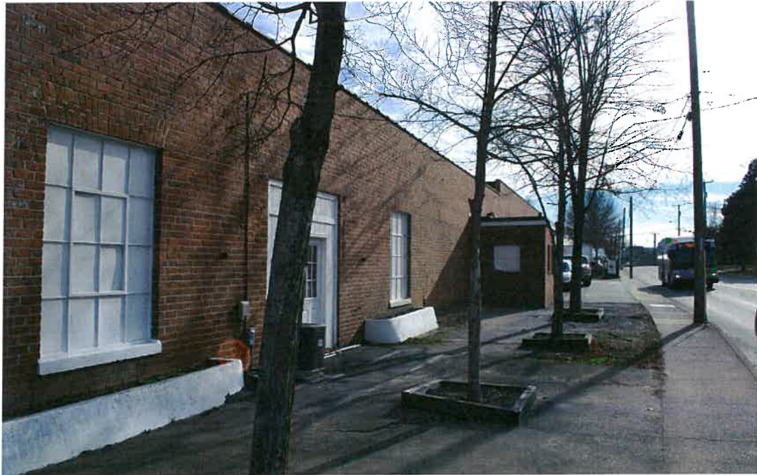
1. DAIRY ELEVATION ALONG 10TH STREET
