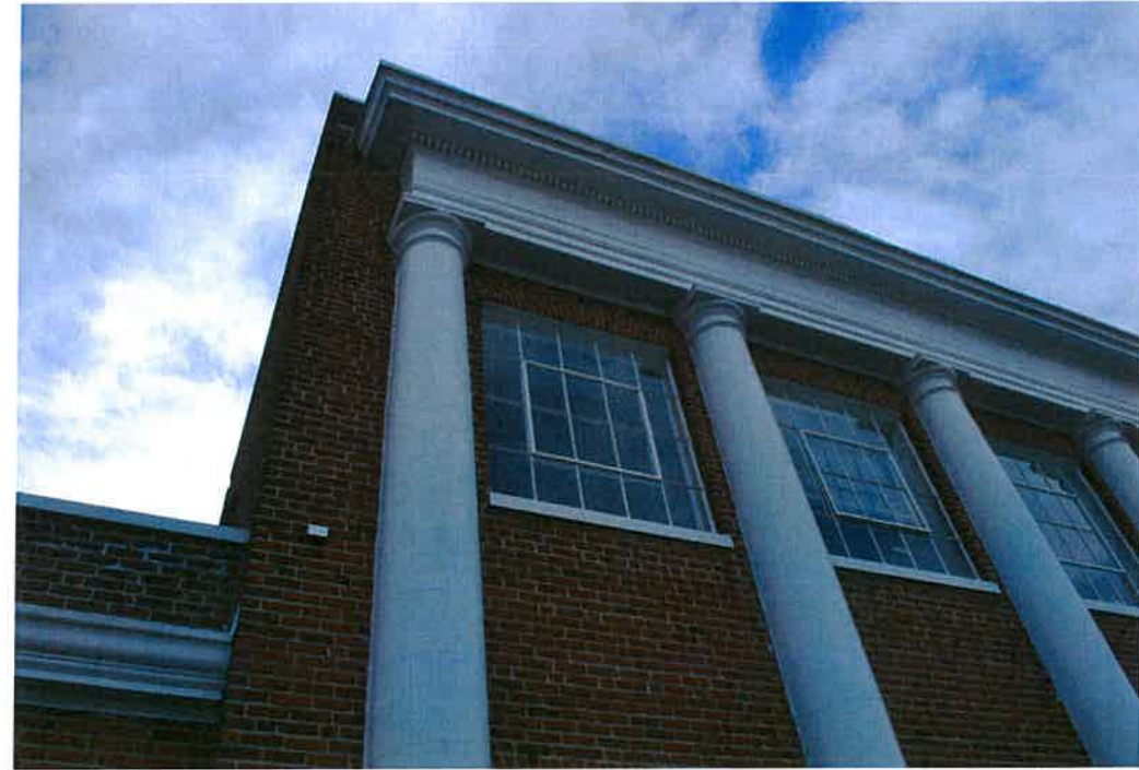
3. DAIRY BUILDING - CORNICE
