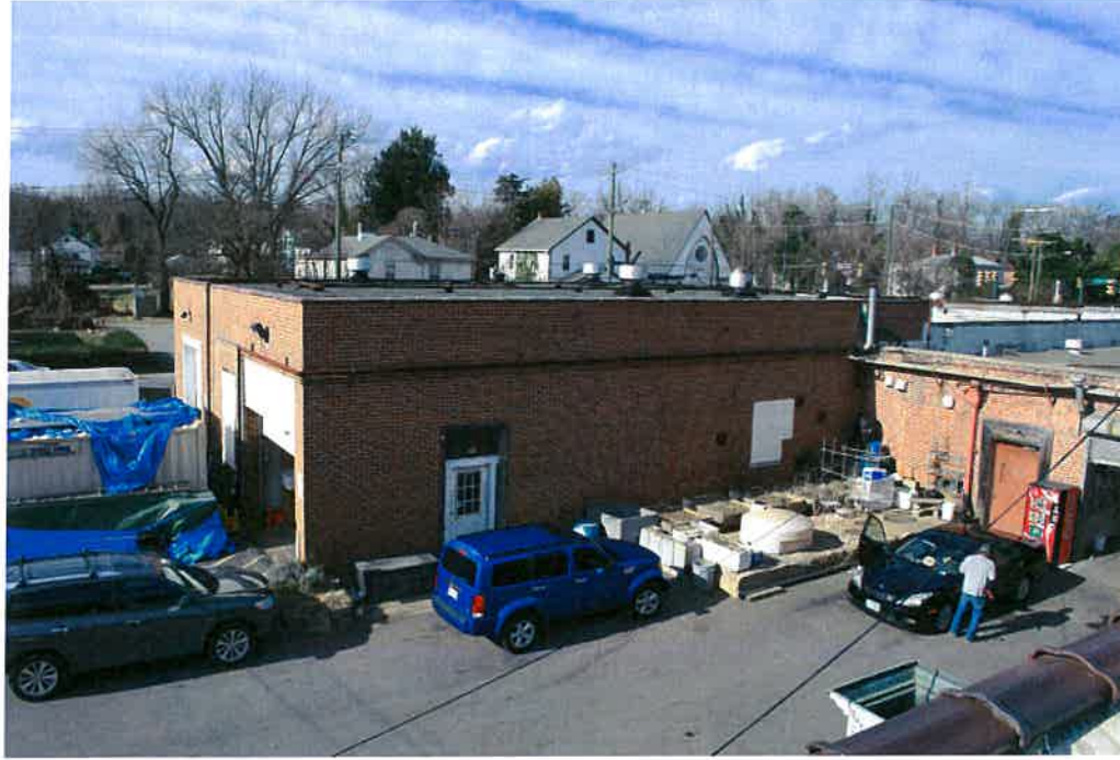
2. DAIRY BUILDING LOOKING TOWARDS 10TH STREET
