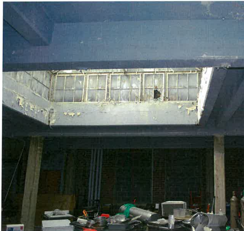
4. EXISTING SKYLIGHT IN DAIRY BUILDING
