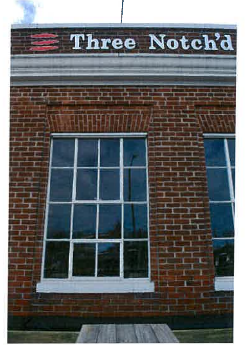
4. DAIRY BUILDING - WINDOW
