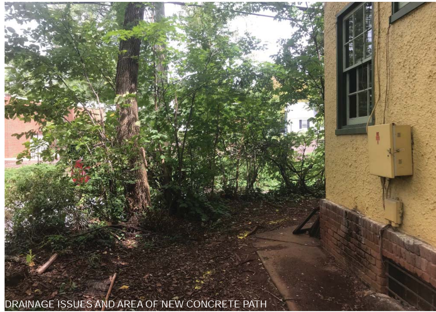
DRAINAGE ISSUES AND AREA OF NEW CONCRETE PATH
