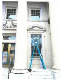
PROPOSED PENDANTS TO HANG @ 134" BELOW EXISTING PORCH CEILING. BLUE TAPE IN PHOTO IS REPRESENTATIVE OF LOCATION AT BOTTOM OF PROPOSED FIXTURE.
