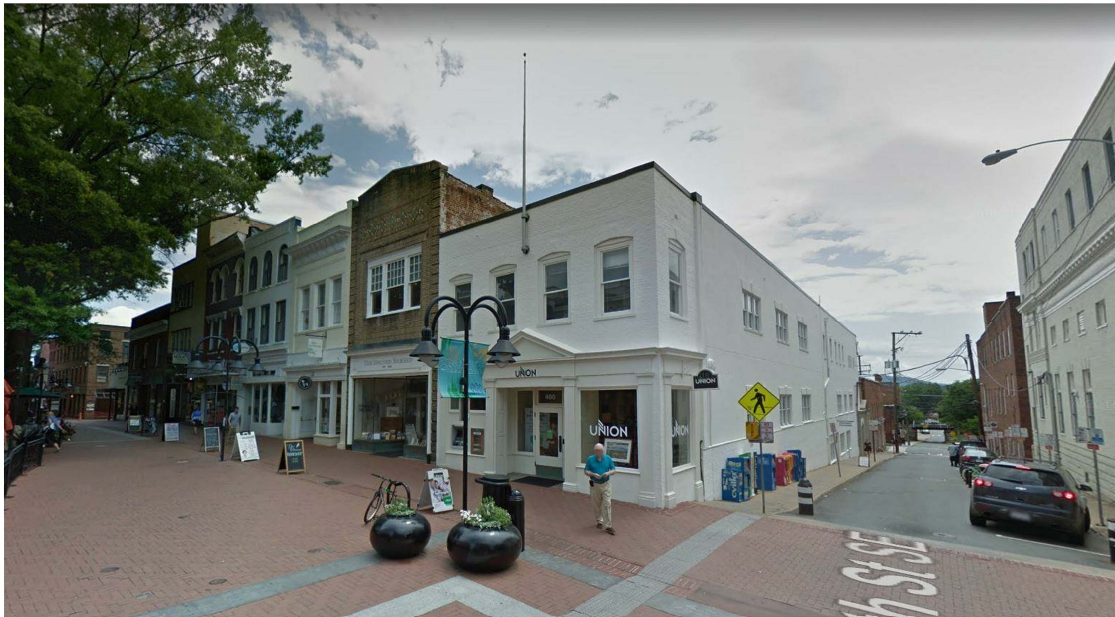
DOWNTOWN MALL SIDE STREET VIEW
