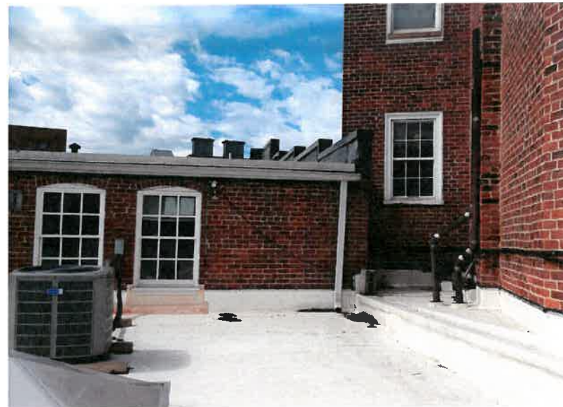
VIEW OF UPPER ROOF FROM MECHANICAL UNITS
