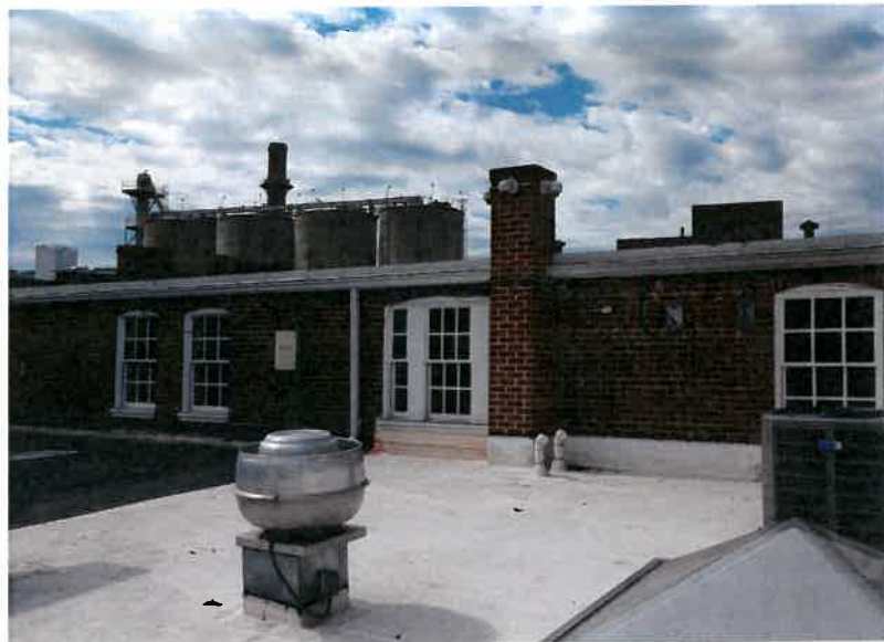
VIEW OF UPPER ROOF FROM MECHANICAL UNITS
