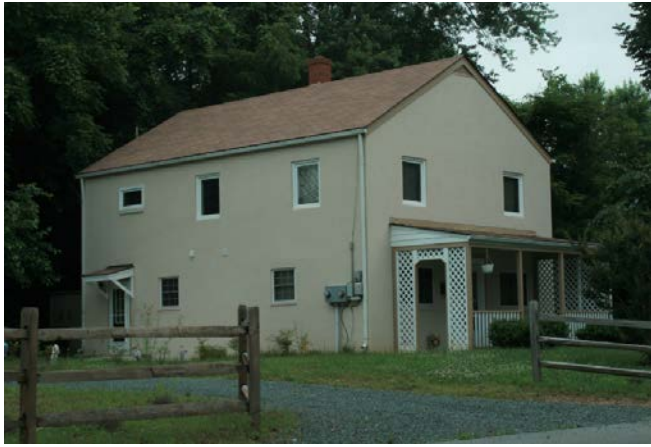
123 Franklin Street (Originally built as a store, c1955.)
