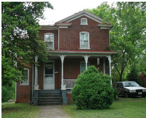
1606 East Market Street
