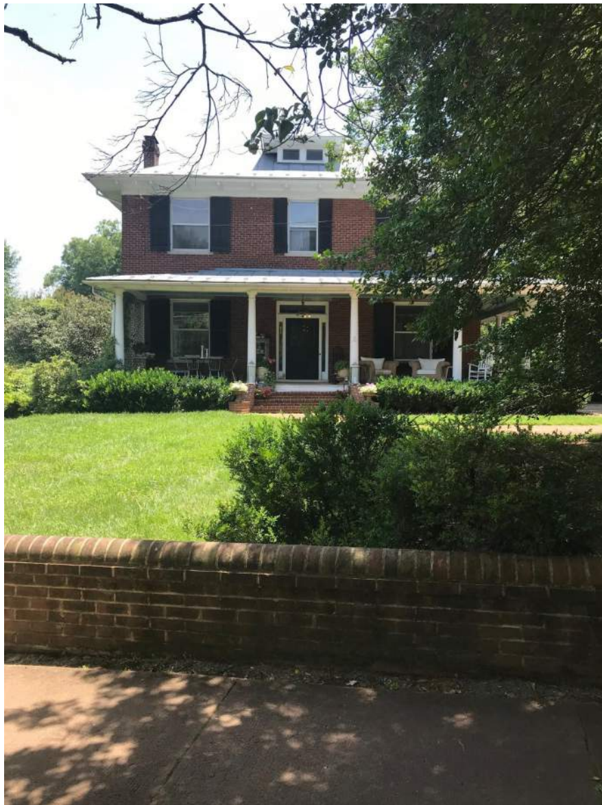
Existing Brick Wall at Front of House
