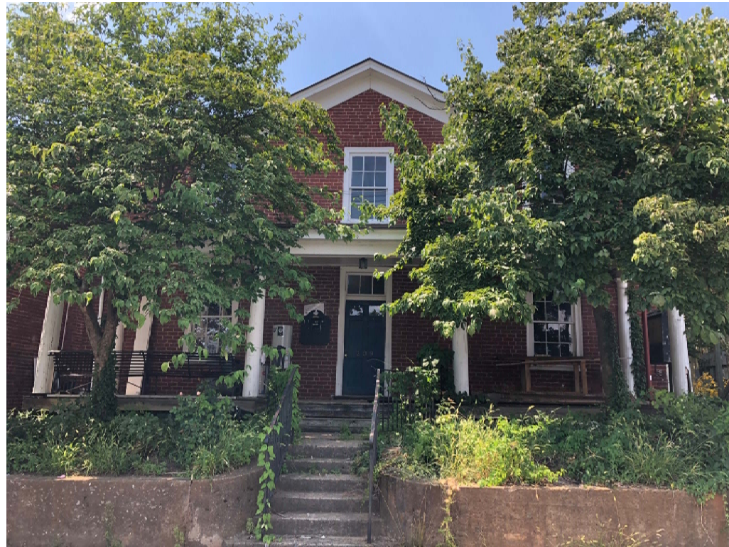
EXISTING - FRONT FROM SIDEWALK
