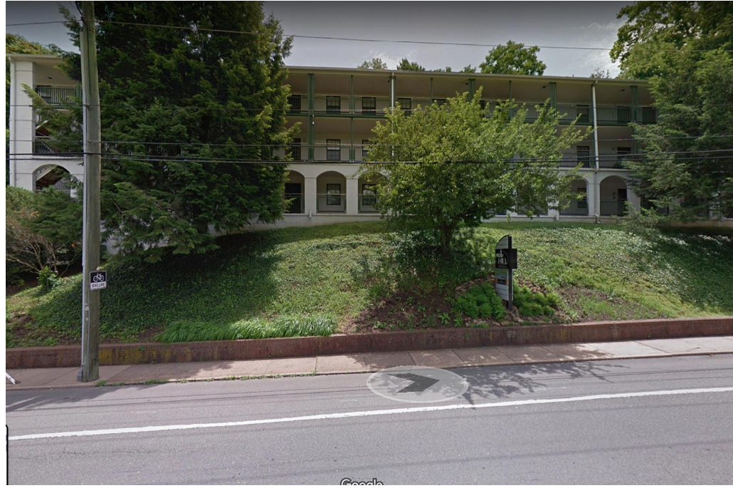
STREET VIEW – ENTIRE BUILDING
