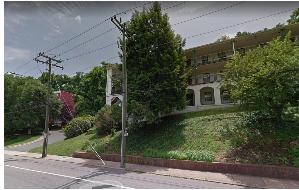
STREET VIEW – LOCATION OF NEW STAIRS
