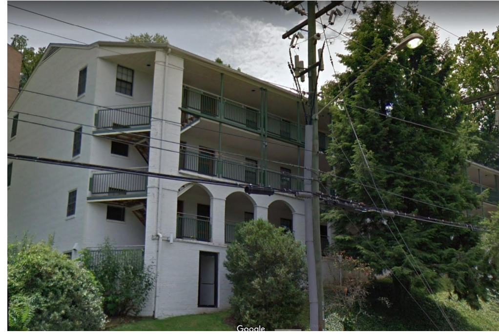
STREET VIEW – EXISTING STAIRS TO BE REPLACED
