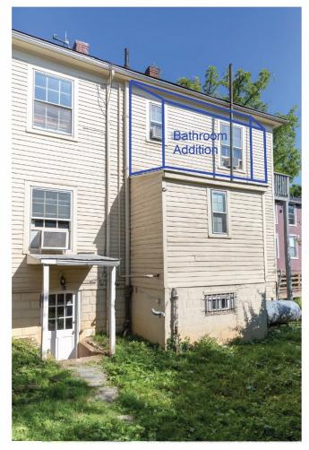
Existing (small) window and trim will be reused in new wall and align with window below.
