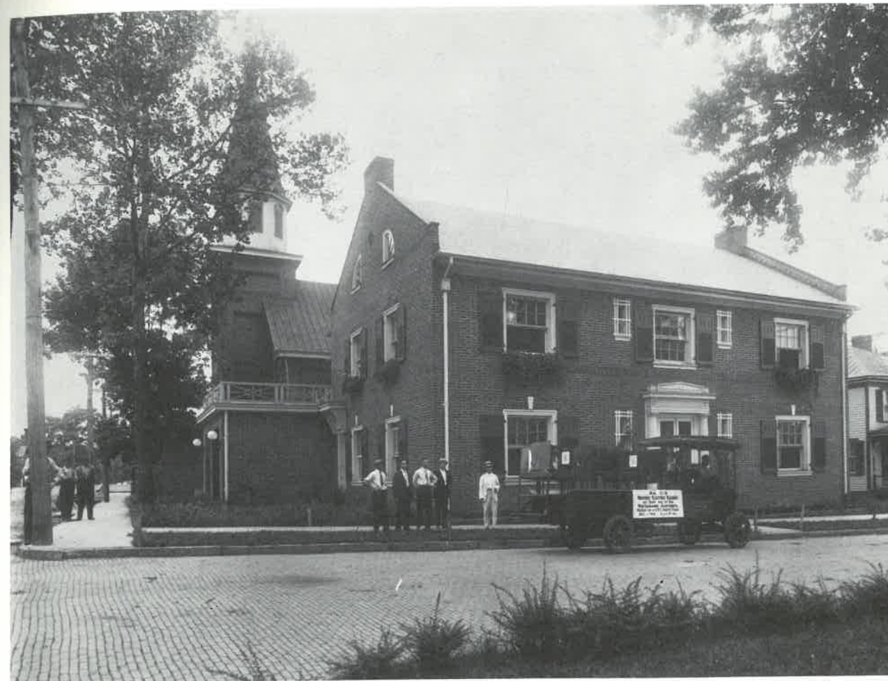
The C & A offices at Ridge and Main about 1 August 1916. The occasion seems to be the shipment of six Hughes electric ranges to the Wertebaker Apartments. Holsinger
